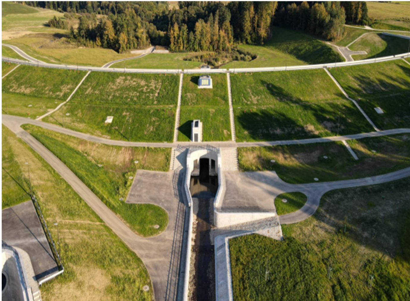
Phot. 4 View of the bottom outlet of the dam.
