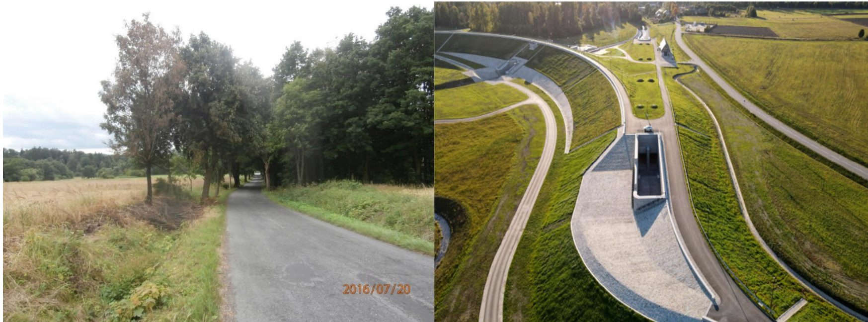
Phot. 3 Section of powiat road no. 3233D running through the area of the right-bank abutment of the dam.
