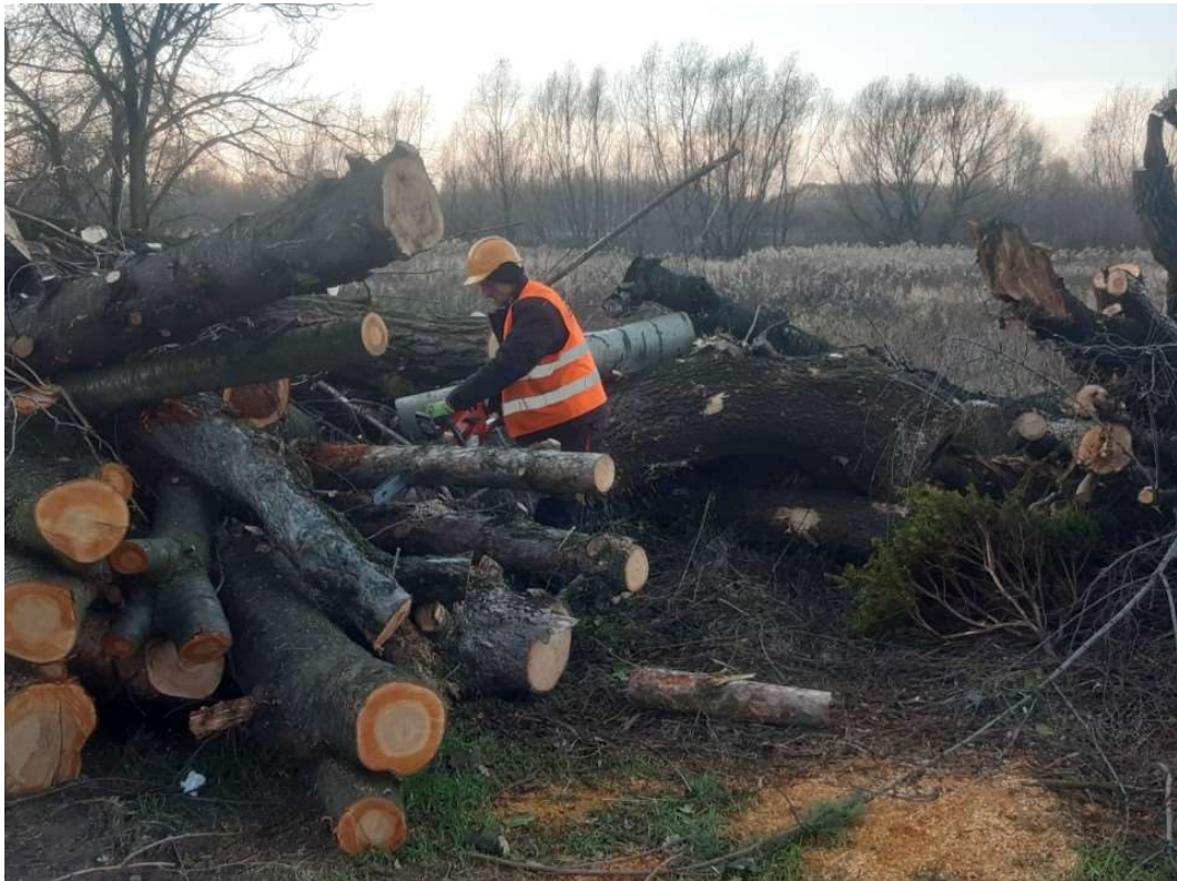
Photo. 10. Tidying-up of the area after removal of trees.
