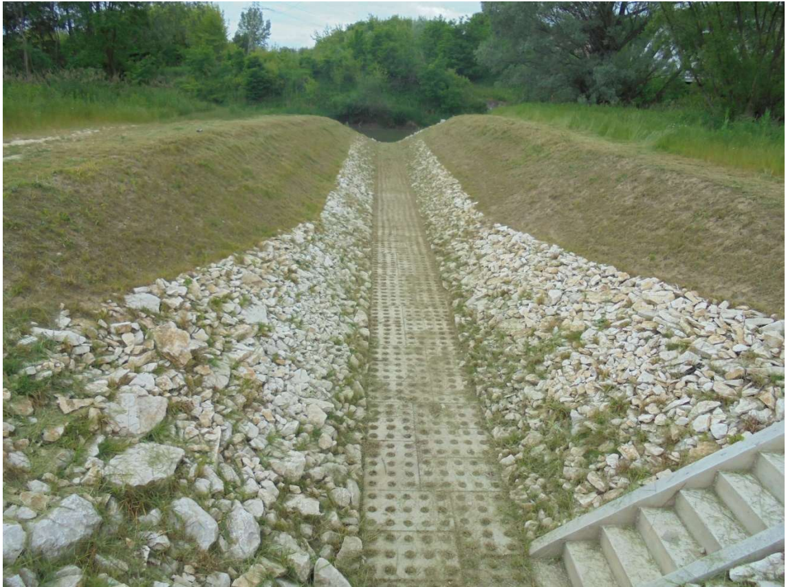
Photo. 25. New embankment of the Biała River after completion of construction.
