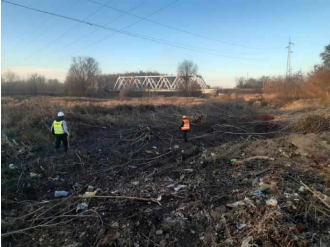
Photo. 9. Removal of trees in the embanked area of the Biala River.
