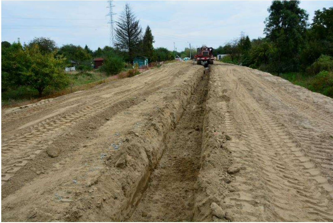
Photo. 20. Excavation for anti-filtering shield, 2nd decade of September 2021.
