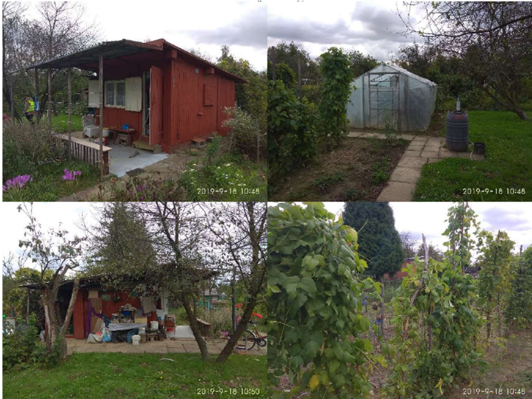
Photo. 5. Condition of the Construction Site before the start of works implementation – allotment gardens at FAG SEMAFOR.
