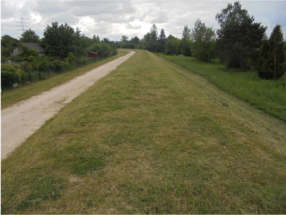
Photo. 24. New embankment of the Biała River after completion of construction.
