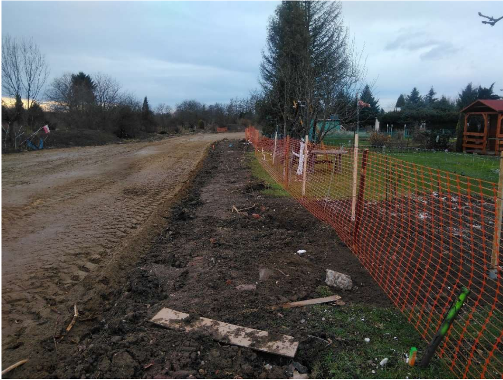
Photo. 15. Fencing off the zone of allotment gardens from the belt of works, 2nd decade of December 2020.
