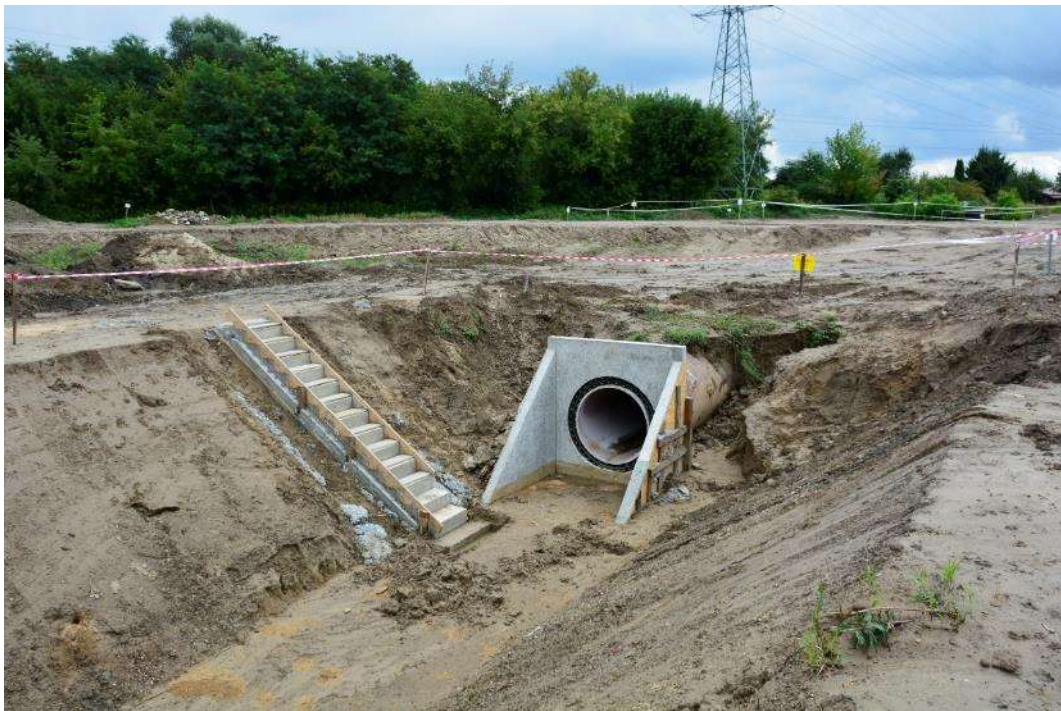
Photo. 19. Excavation area for the storm sewer, 3rd decade of August 2021.
