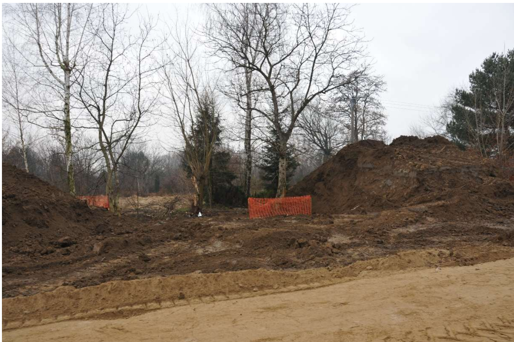
Photo. 14. Construction of embankment, 2nd decade of December 2020.
