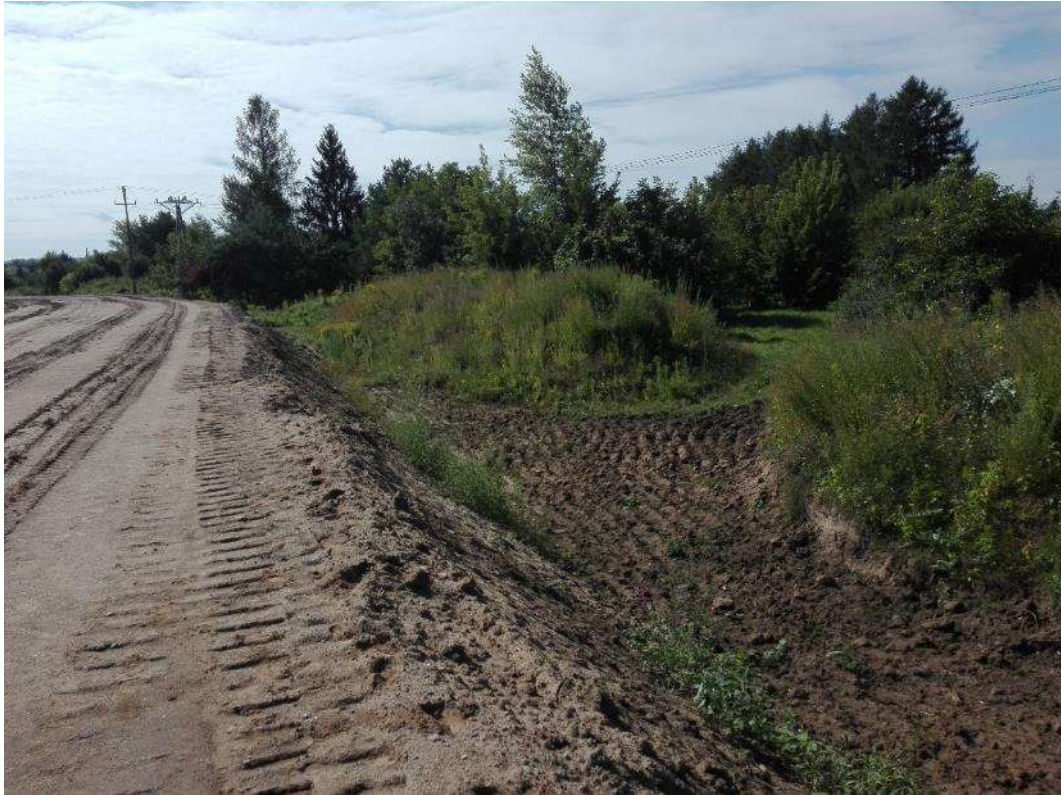
Photo. 18. Construction of embankment, 2nd decade of August 2021.
