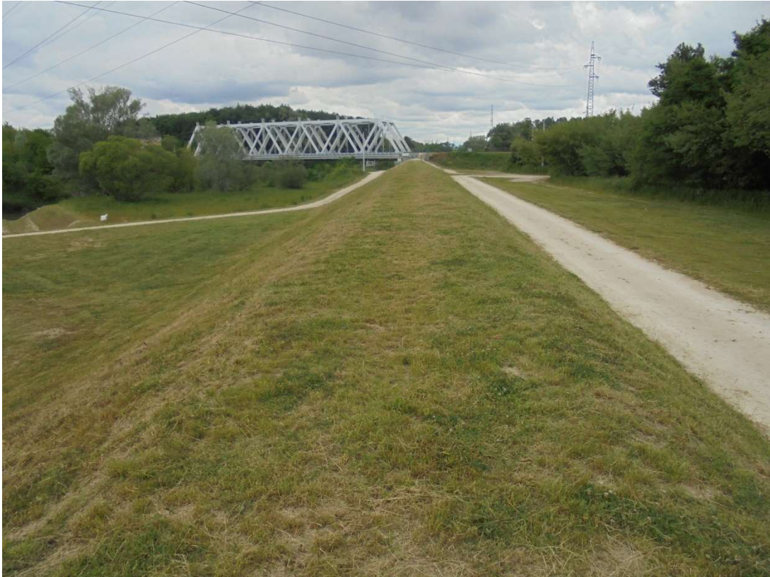
Photo. 23. New embankment of the Biała River after completion of construction.
