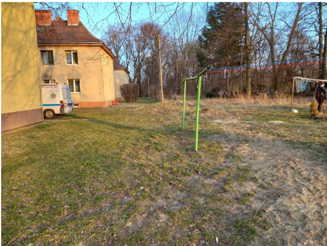
Photo. 9. Condition of the site before the start of construction - construction of the teletechnical network along the distance of the sluice channel of the Przewóz barrage, status in the third decade of March 2022 (view towards the east).
