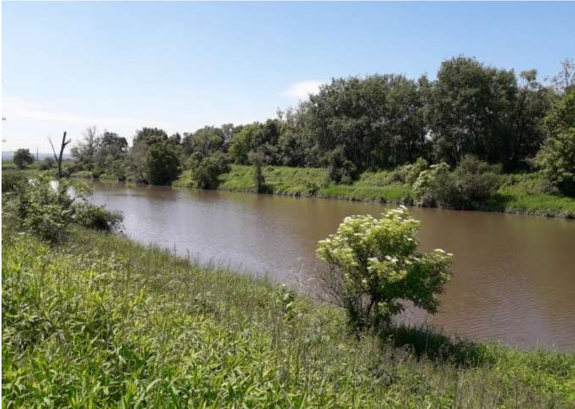
Photo. 3. Condition of the site before the start of construction – view in the location of the flood gate.
