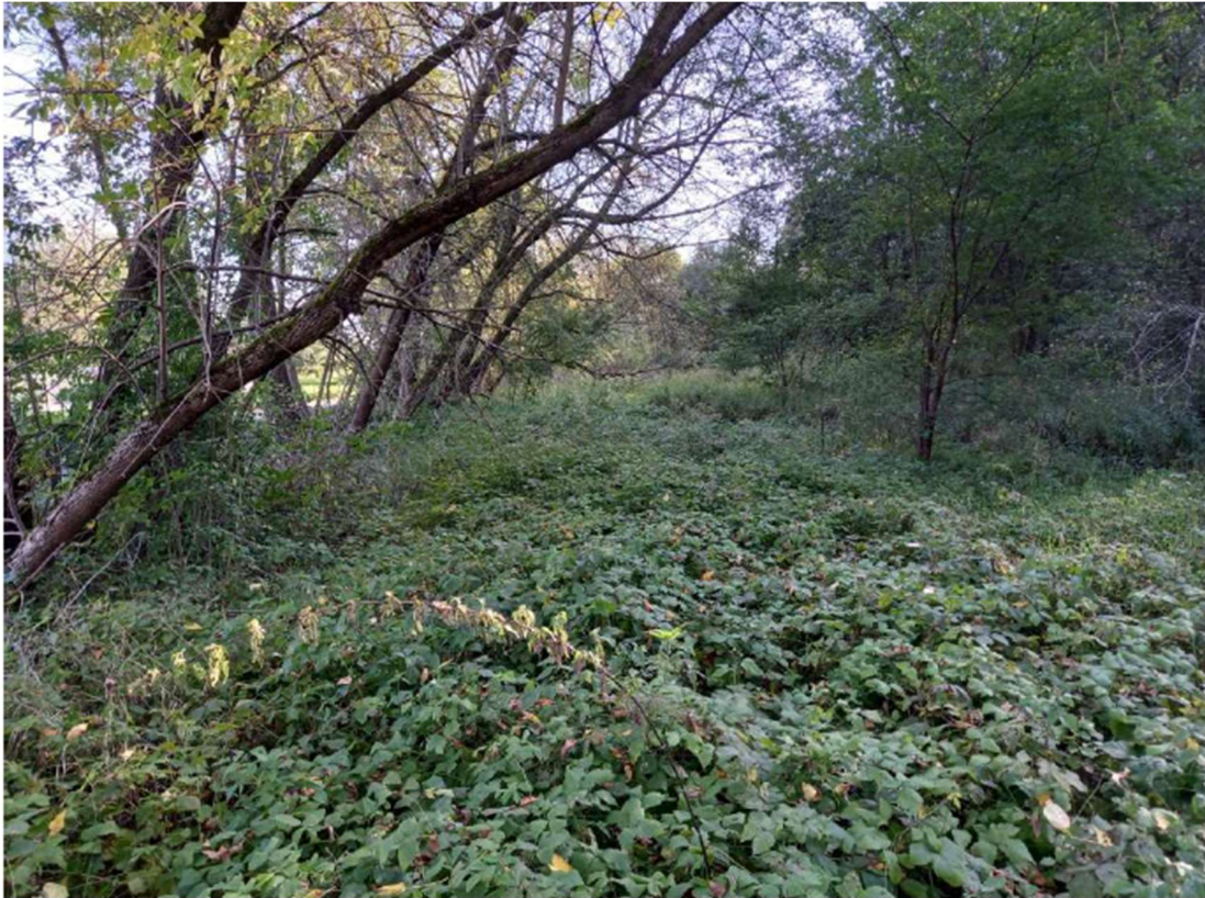
Photo. 37. Site after the construction of the power network at the distance along Dymarek Street, status in the third decade of September 2023 (view towards the south).
