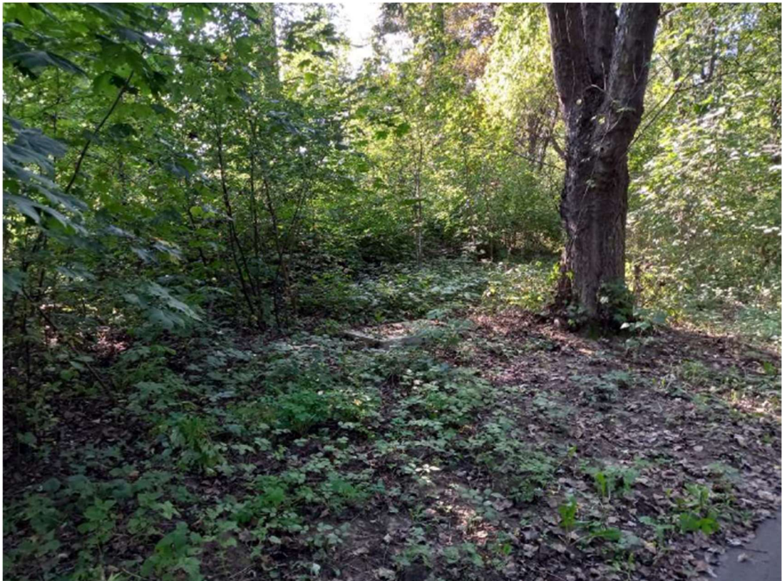
Photo. 38. Construction site of the teletechnical network at the distance along the sluice channel of the Przewóz barrage, status in the third decade of September 2023 (view towards the west).
