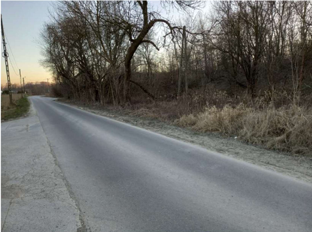
Photo. 7. Condition of the site before the start of construction - construction of the power network along Dymarek Street, status in the third decade of March 2022 (view towards the south).
