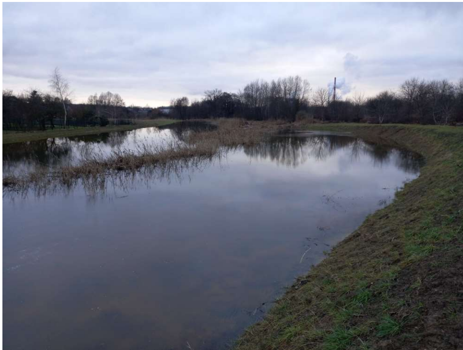
Photo. 52. Condition of the construction site in the last month of the execution of works – the reconstructed reservoir at Ditch 2, western part, status in the third decade of January 2023 (view towards the west).
