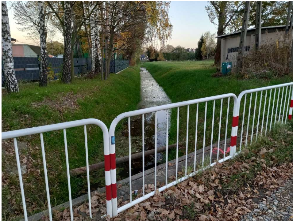
Photo. 38. Growth of grass on bank slopes at Ditch 2 after finishing the works at this section, (view towards the east).
