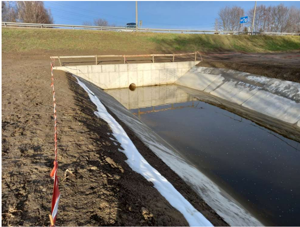
Photo. 23. Protection of hazardous places on the construction site of the embankment sluice at Ditch 2a at the embanked area of the Vistula, status in the third decade of December 2022 (view towards the north).
