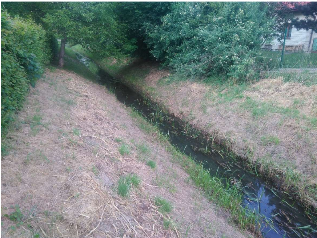
Photo. 4. Condition of the site before the start of construction – bed of the Lesisko channel.
