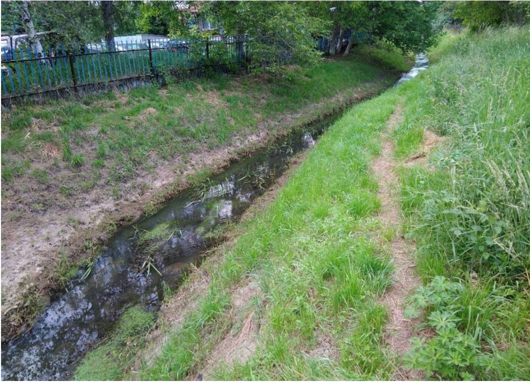
Photo. 3. Condition of the site before the start of construction – bed of the Lesisko channel.
