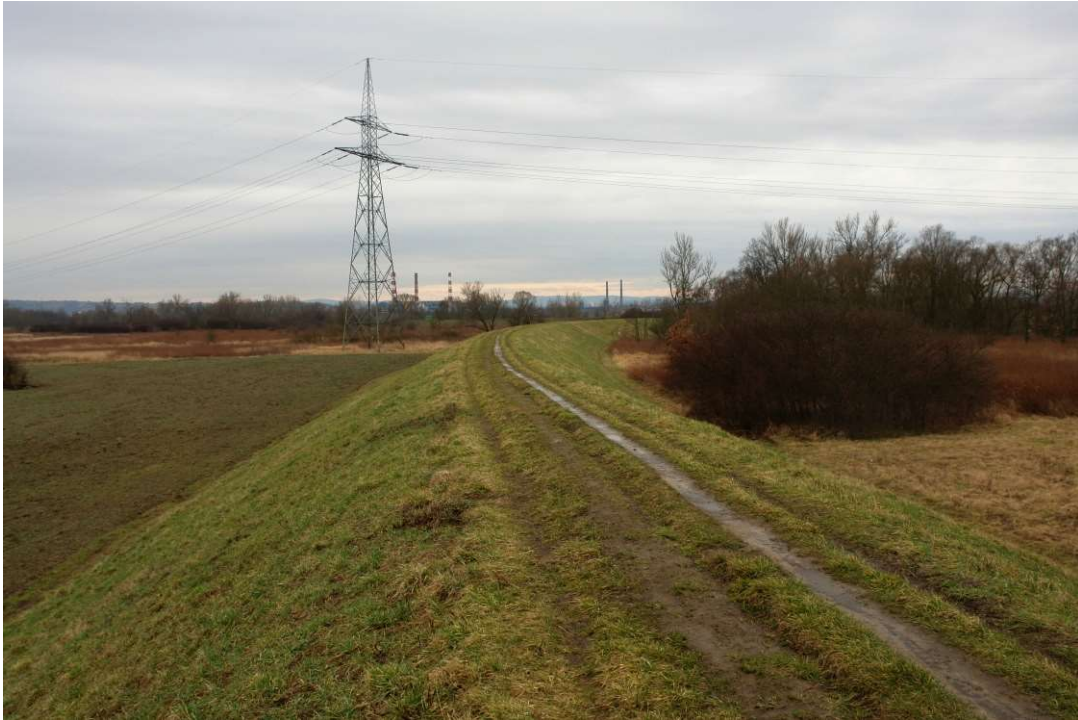
Photo. 1. Condition of the Construction Site before the start of works - the right embankment of the Vistula River planned for reconstruction for Task 1, the condition in the third decade of February 2020 (upstream view).
