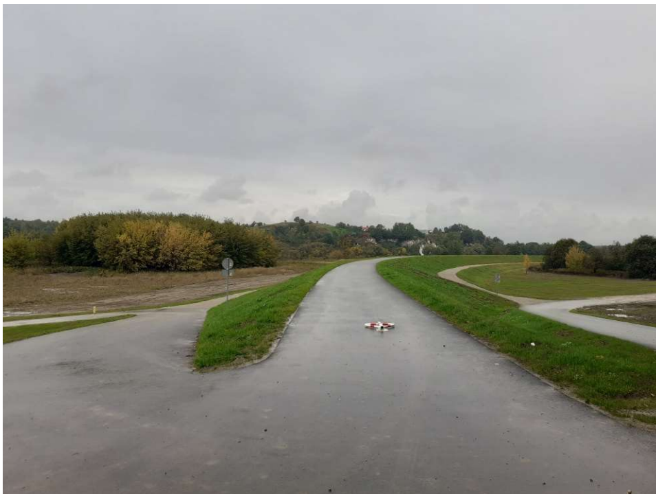
Photo. 45. Reclaimed area of the former operating backyard (after the end of temporary occupation) on the right-bank area beyond the embankment of the Vistula River along Task 2, condition in the third decade of September 2022 (downstream view).
