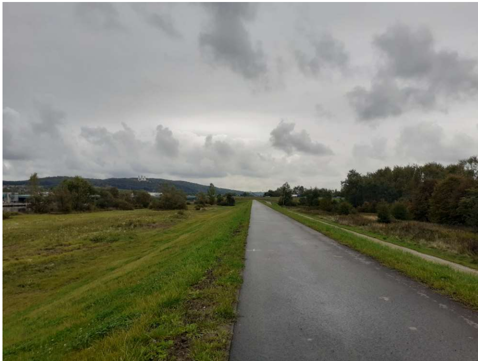
Photo. 43. Condition of the construction site in the last month of the period of execution of works – the right embankment of the Vistula River for Task 3, condition in the third decade of September 2022 (downstream view).
