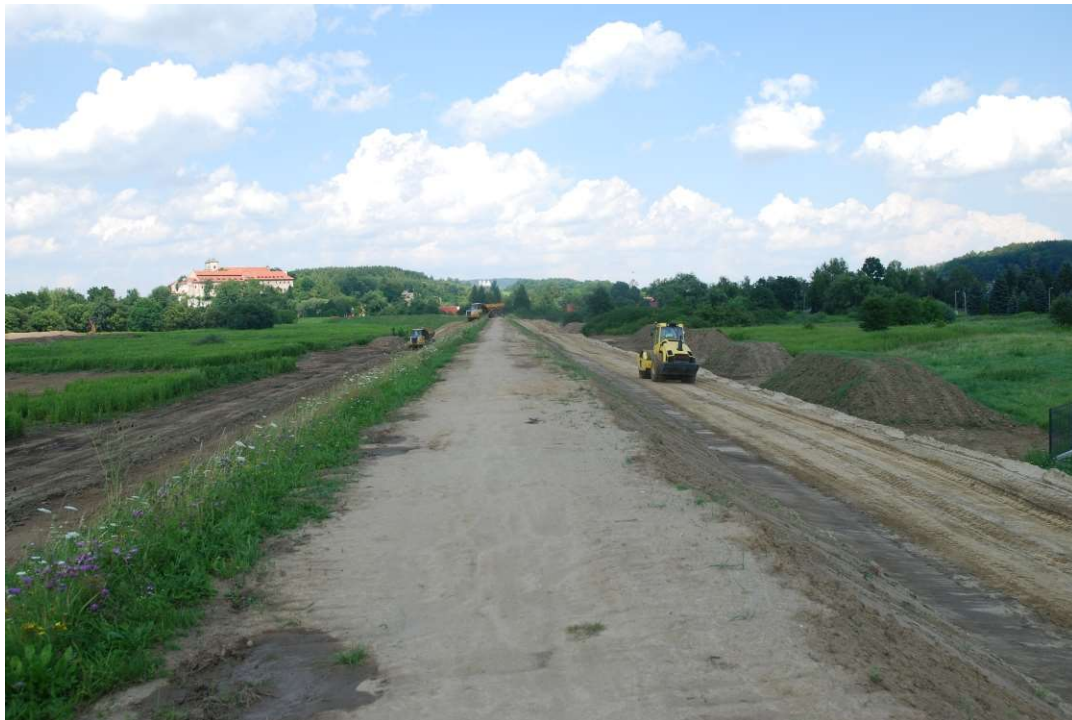
Photo. 21. Protection of the topsoil piles for Task 2, condition in the third decade of July 2020 (downstream view).
