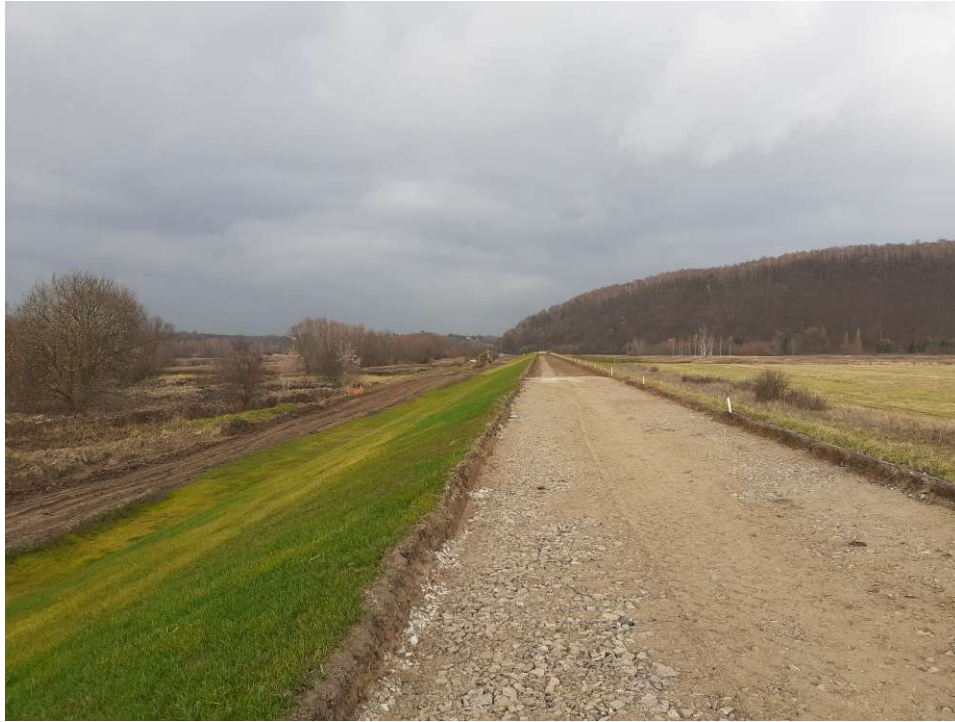
Photo. 36. Growth of grass sown on the flood protection embankment slope for Task 1, condition in the third decade of November 2021 (downstream view).
