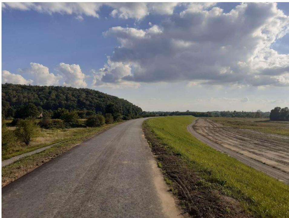
Photo. 37. Growth of grass sown on the flood protection embankment slope for Task 2, condition in the third decade of August 2022 (upstream view).
