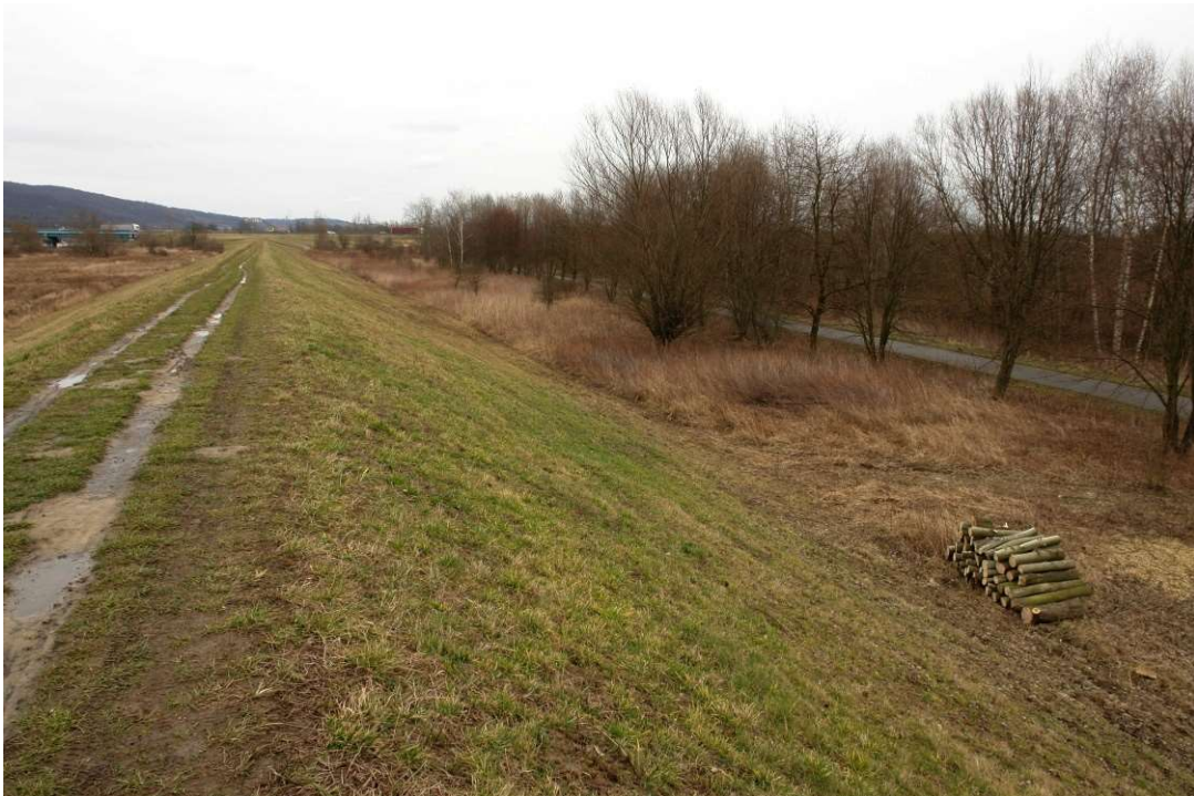
Photo. 8. Condition of the Construction Site before the start of works - the right embankment of the Vistula River planned for reconstruction for Task 3, the condition in the third decade of February 2020 (downstream view).
