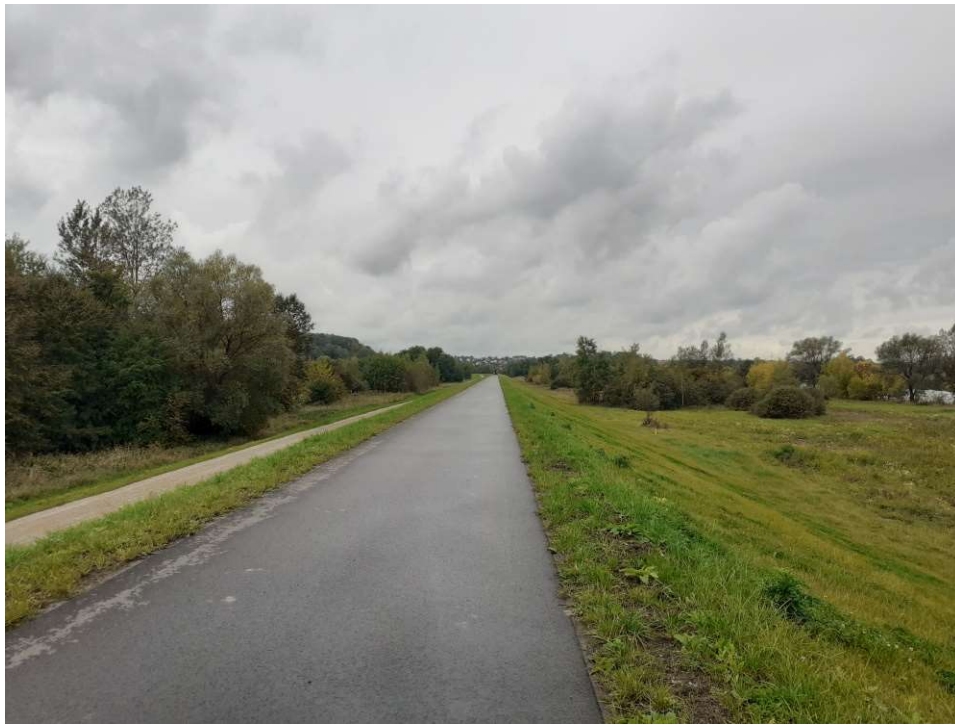
Photo. 42. Condition of the construction site in the last month of the period of execution of works – the right embankment of the Vistula River for Task 3, condition in the third decade of September 2022 (upstream view).
