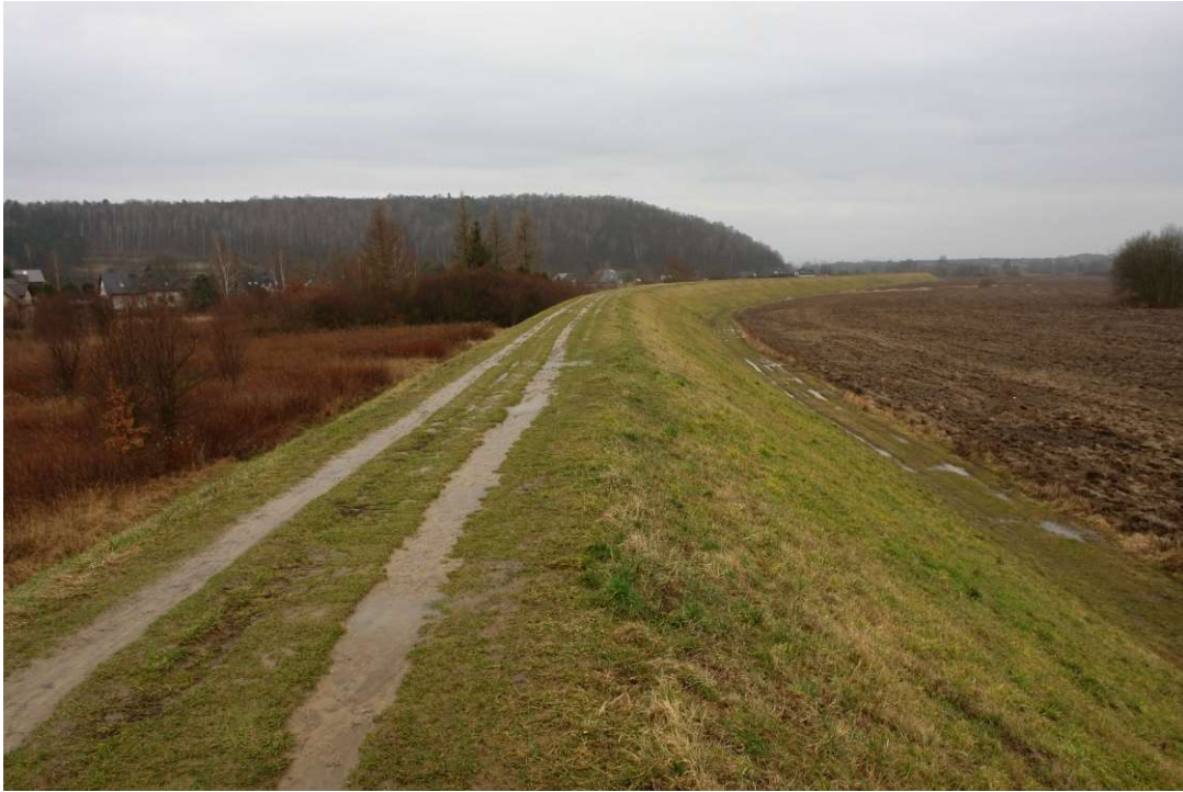
Photo. 5. Condition of the Construction Site before the start of works - the right embankment of the Vistula River planned for reconstruction for Task 2, the condition in the third decade of February 2020 (upstream view).
