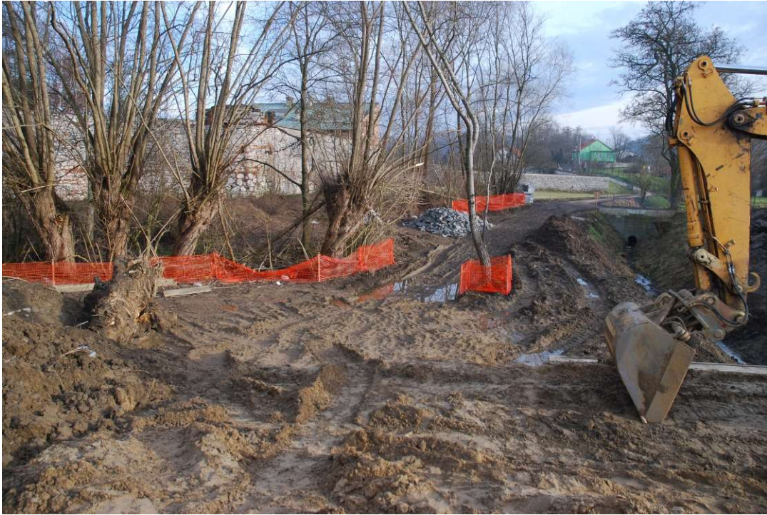
Photo. 16. Protection of trees and bushes not planned for removal for Task 2, condition in the third decade of December 2020 (view towards the area beyond the embankment).
