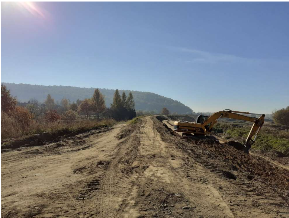
Photo. 33. Topsoiling of slopes of the flood protection embankment for Task 2, condition in the third decade of October 2021 (upstream view).
