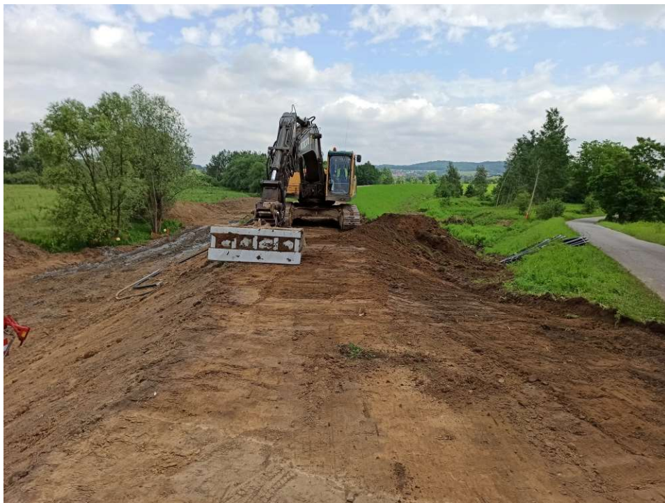
Photo. 19. Removal of the topsoil layer for Task 3, condition in the third decade of June 2020 (downstream view).
