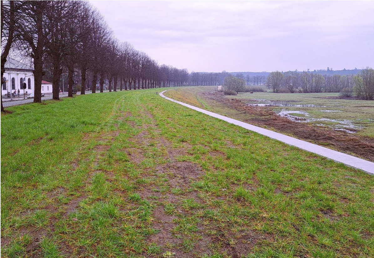
Photo 1 Extended existing embankment
