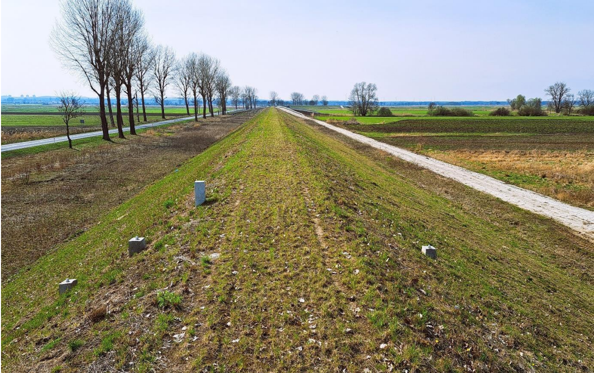
Photo 5 Newly constructed ring embankment
