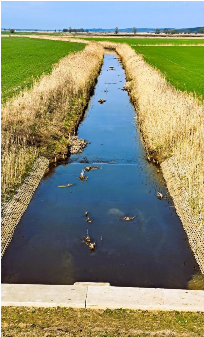
Photo 7 Reconstructed Racza Struga canal
