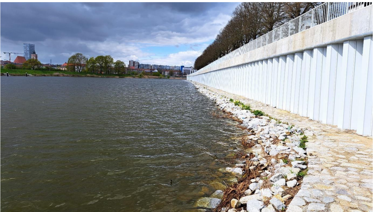
Photo 2 Extended existing embankment
