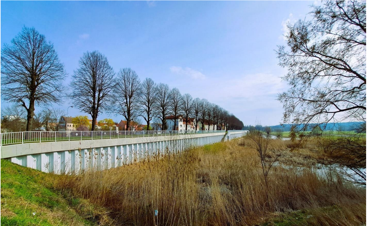
Photo 3 Extended existing embankment
