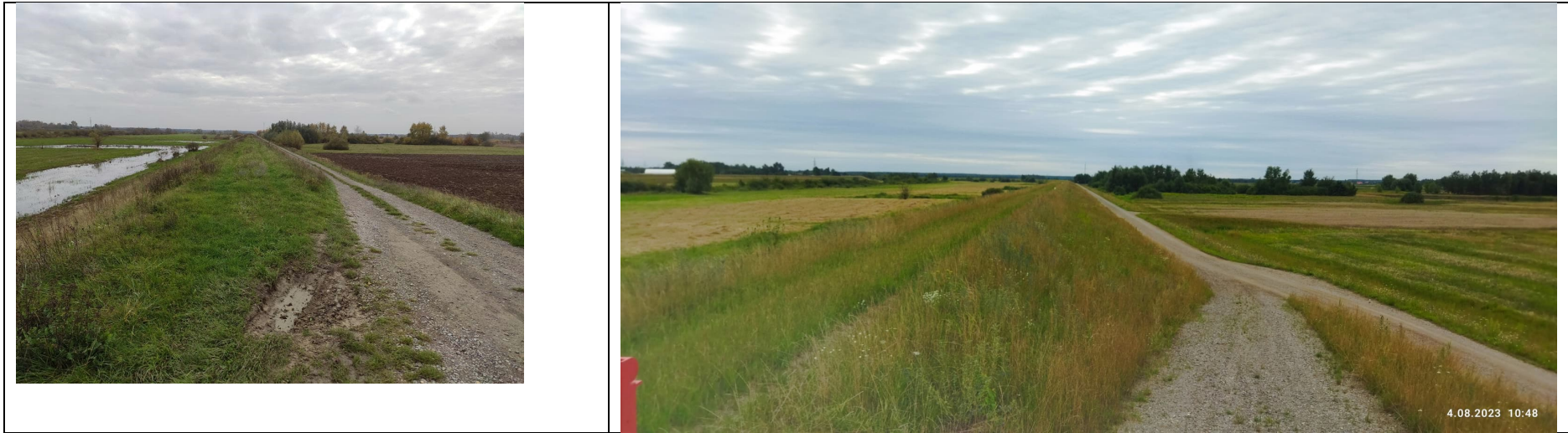
Photo no. 8: Surface water in the embanked area, embankment, road by the embankment on the downstream side.
