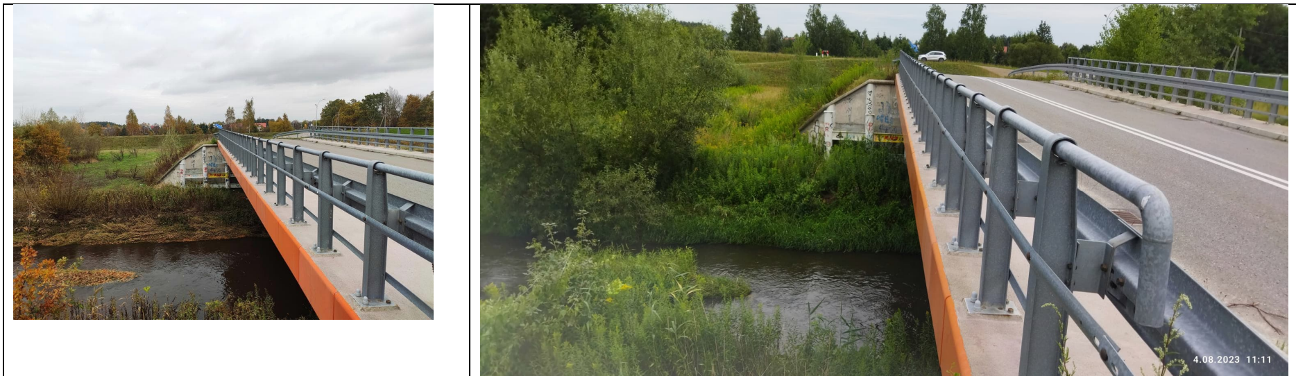
Photo no. 1: Bridge over the Łęg River, Orliśka – Gorzyce road.
