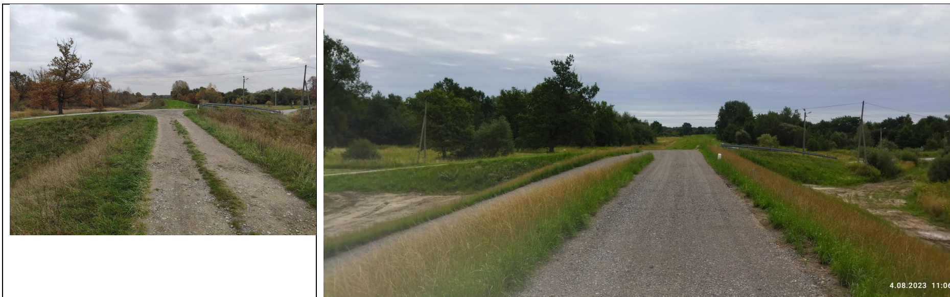
Photo no. 12: End of investment – Orlińska – Gorzyce road.
