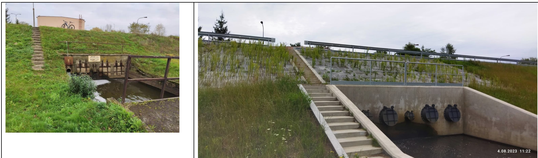
Photo no. 8: Rainwater outflow, treatment plant building in the distance.
