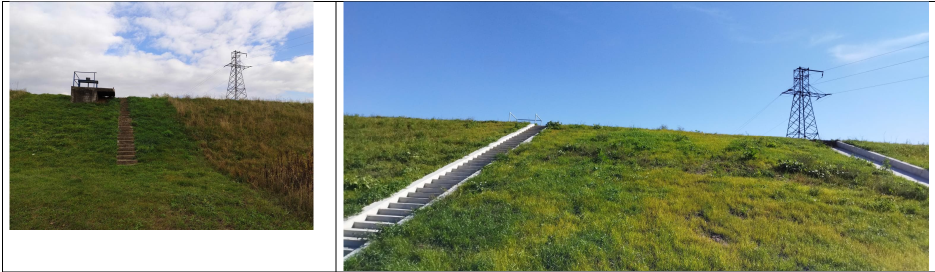
Photo no. 21: Embankment culvert, gate valve, HV line.
