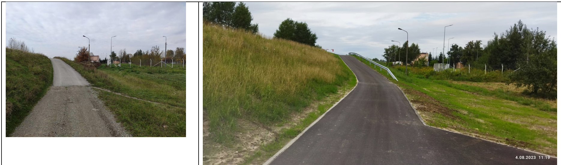
Photo no. 5: Entrance to the embankment at the treatment plant (asphalt surface).
