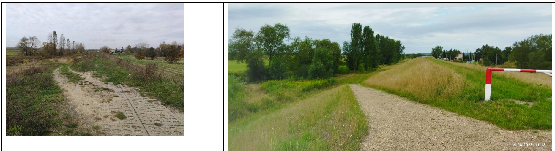
Photo no. 4: Reinforcement of the crossing across the embankment.
