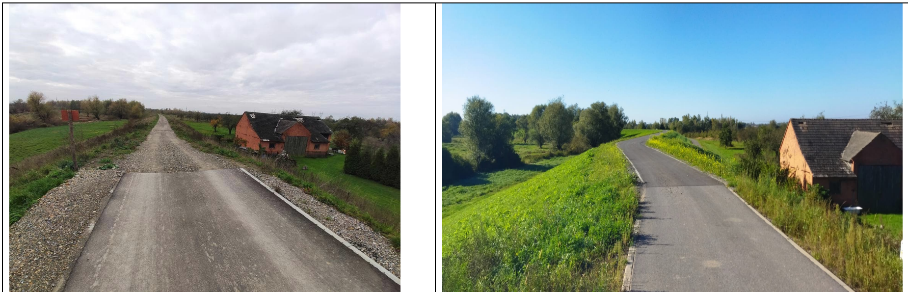
Photo no. 1: Start of left-side embankments, utility building.
