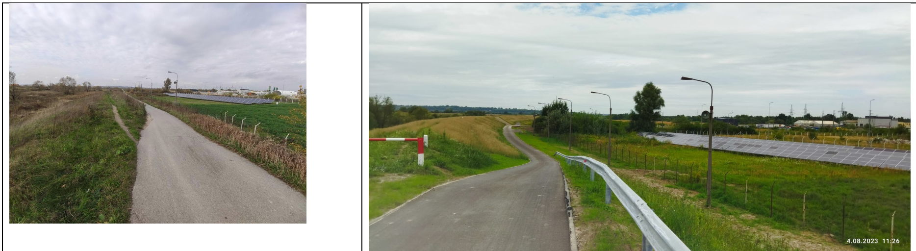
Photo no. 9: Asphalt road exit from the embankments, photovoltaic farm in the distance.
