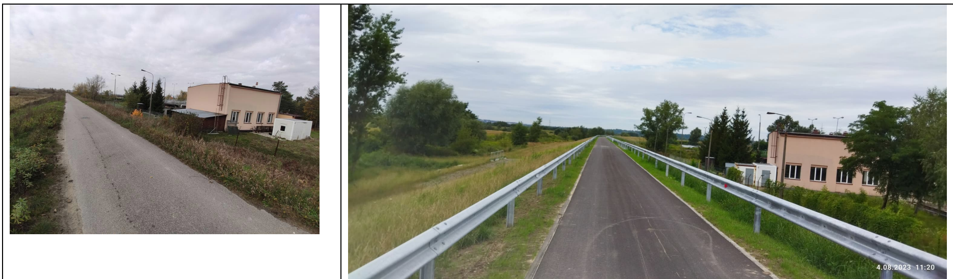
Photo no. 6: Treatment plant buildings.
