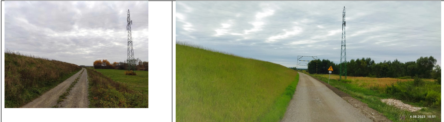
Photo no. 9: Embankment, gravel road, HV line, adjacent areas.
