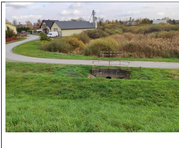
Photo no. 16: Culvert under Podwale Street.
