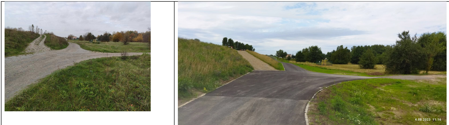
Photo no. 3: Road junction with entrance to embankments, gas reduction station in the distance.
