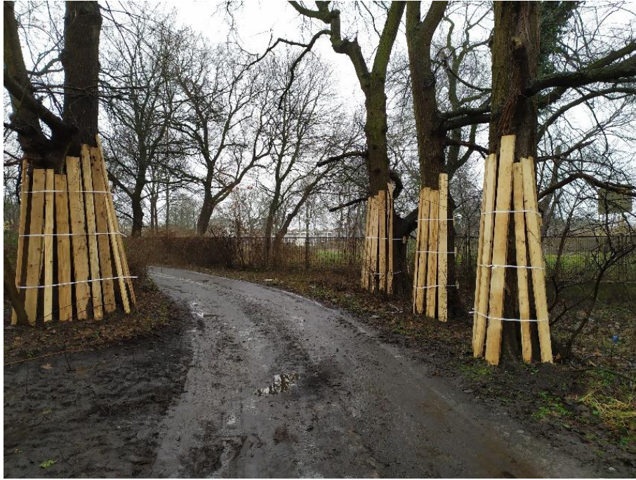
Photo 3. Protection for trees at risk of damage.
