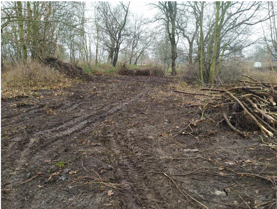
Photo 2. Tree and shrub felling in the Task area.
