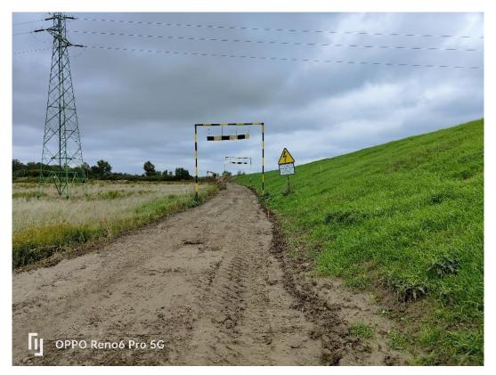
Phot. 32. View of the right embankment at km approx. 4+100 – gate structures - protection zones under the active power line, September 2022
