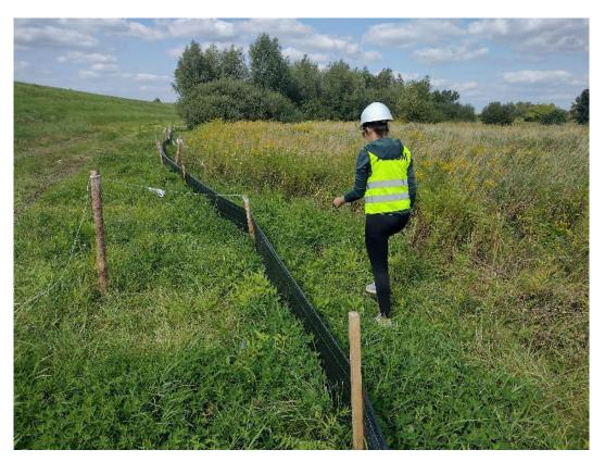
Phot. 9. View of the left embankment at km approx. 1+700 – inspection of the implementation status of herpetological fences, August 2021
