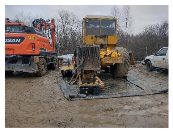
Phot. 6. View of the right embankment at km approx. 2+400 – site facilities – sealing of the subbase under serviced machines, January 2022
