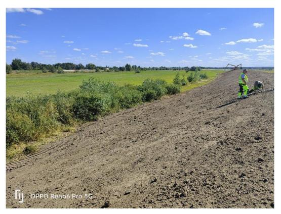
Phot. 25. View of the left embankment at km approx. 2+400 – spreading the topsoil after executing the embankment extension works, September 2022
