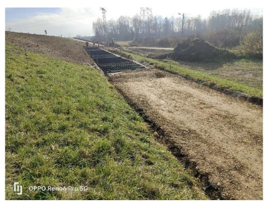
Phot. 31. View of the left embankment at km approx. 1+100 - view of hardening works for service roads, November 2022
