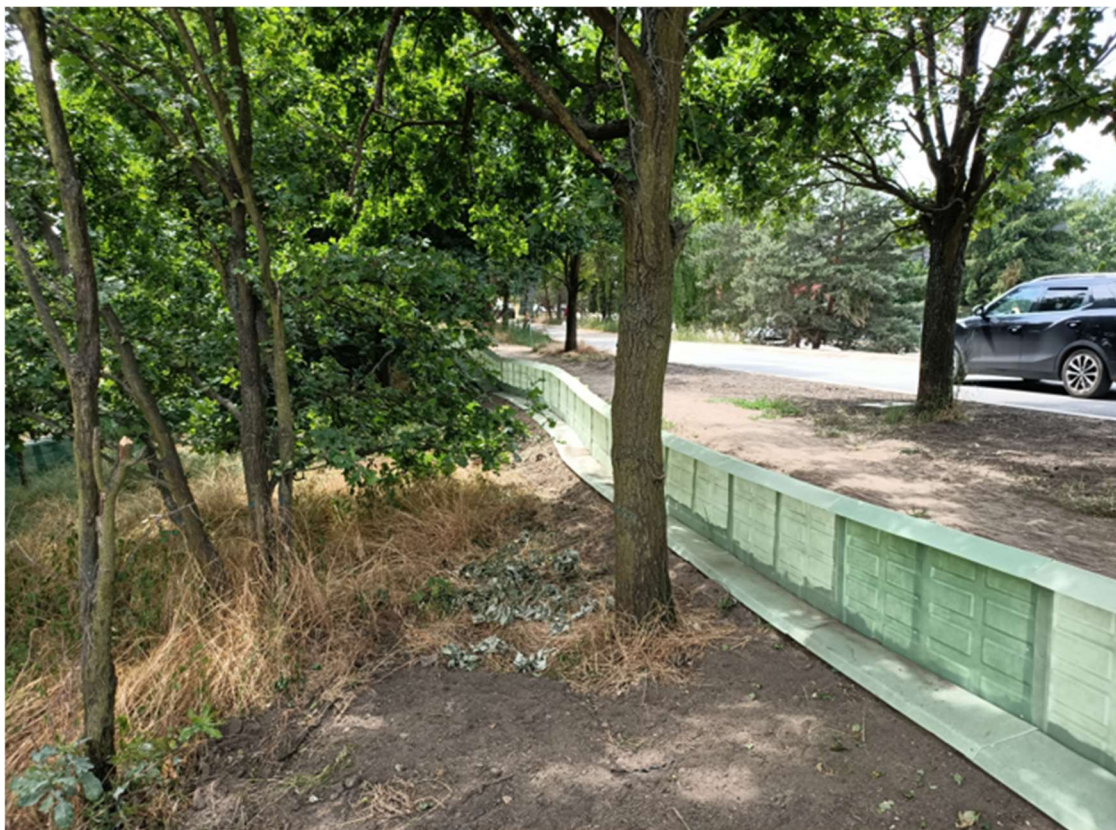
Foto. 9. Ślężoujście Street , third decade of June 2023 (fencing installed along Potokowa Street).
