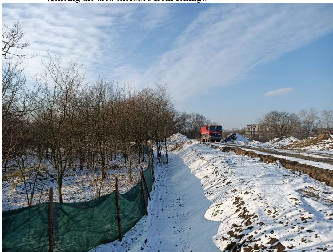
Foto. 4. Ślężoujście Street , second decade of December 2022 (fencing of the Construction Site).
