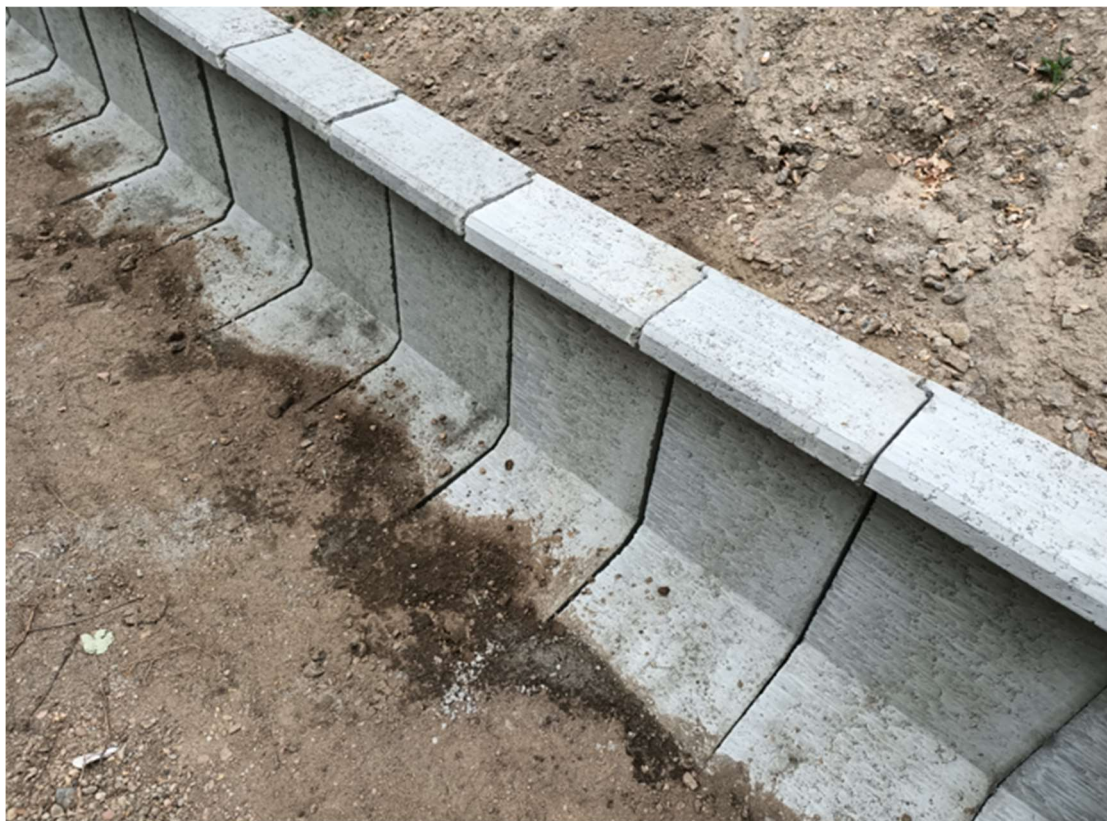
Foto. 7. Ślężoujście Street , second decade of June 2023 (installation of permanent herpetological fencing at the foot of the slopes).
