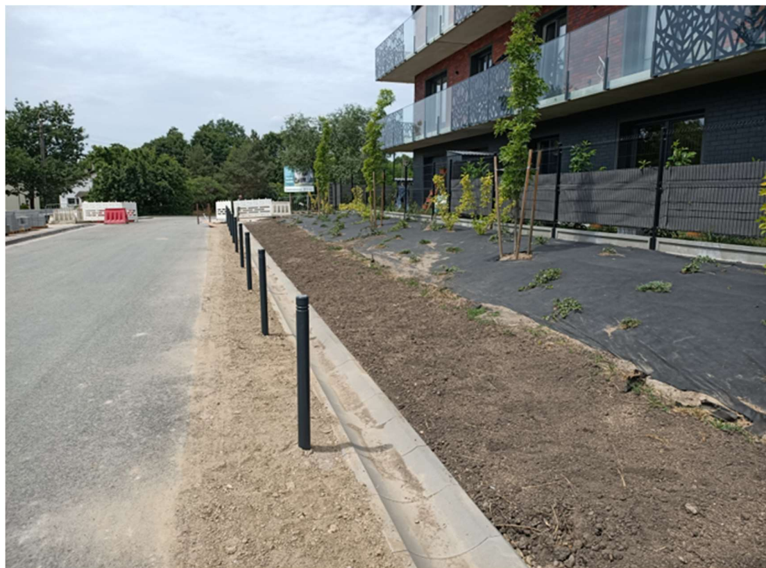
Foto. 8. Ślężoujście Street , first decade of June 2023 (completed road works, tidied roadside).
