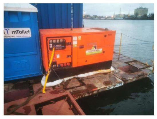
Photo 9 Power generator with additional spill protection on a vessel
