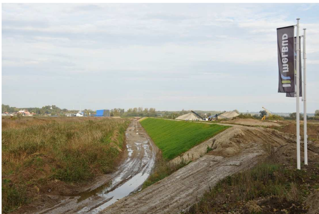
Fig. 44. Growth of grasses sown on the slope of the flood embankment – right bank of Koprzywianka river downstream of the bridge on the road Szewce-Skotniki, status in the third decade of October 2020 (downstream view).
