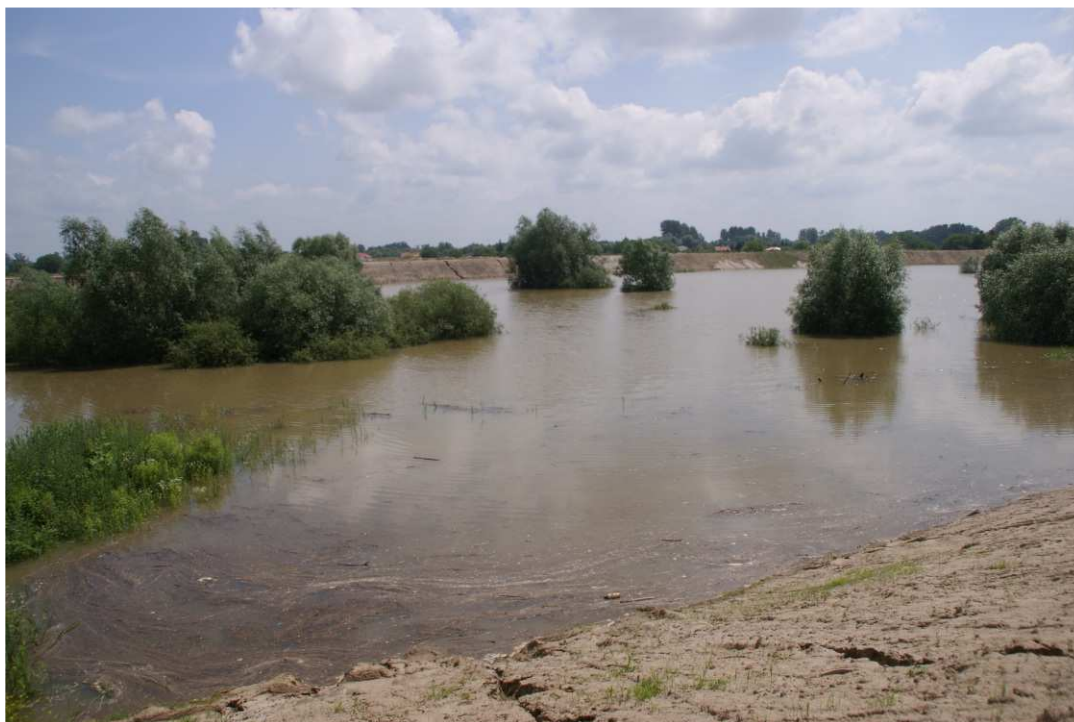
Fig. 47. Flooding from Koprzywianka in the area of works – banks of Koprzywianka river upstream of the bridge on the road Sandomierz-Zawisłecze, status in the third decade of June 2020 (upstream view).
