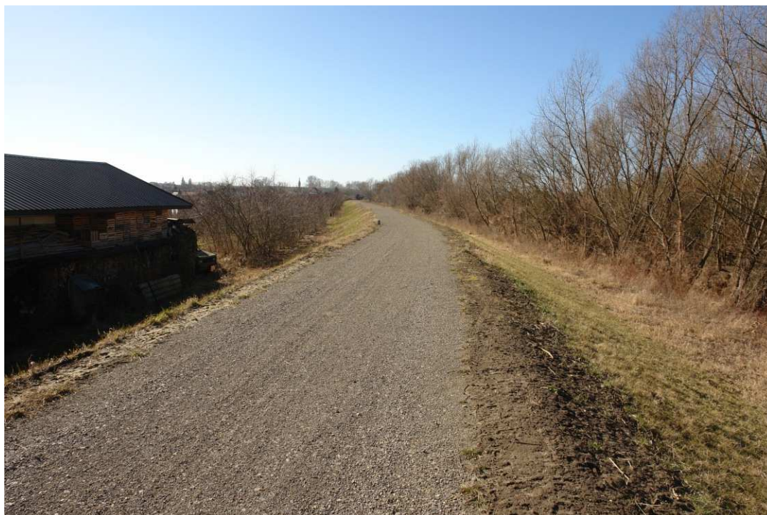
Fig. 55. Site condition in the last quarter of the works implementation period on Task 4 – right bank of Koprzywianka river upstream of the footbridge in Koprzywnica, status in the third decade of February 2022 (upstream view).
