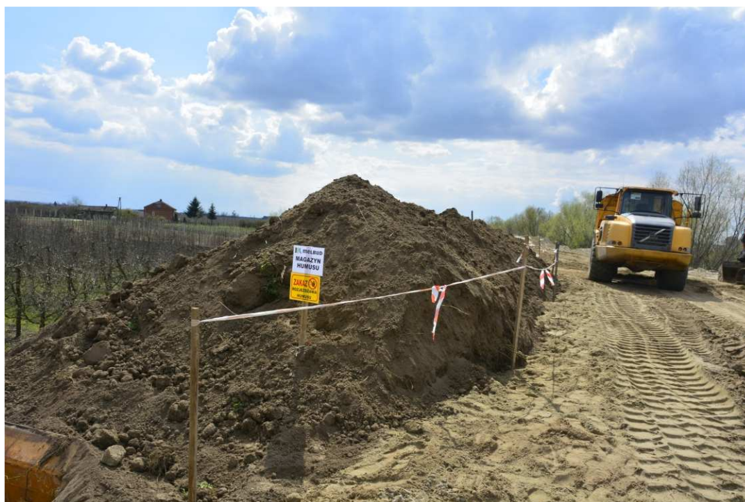
Fig. 24. Protection of top-soil piles – right bank of Koprzywianka river upstream of the bridge on the road Sońniczany-Skotniki, status in the second decade of April 2021 (upstream view).
