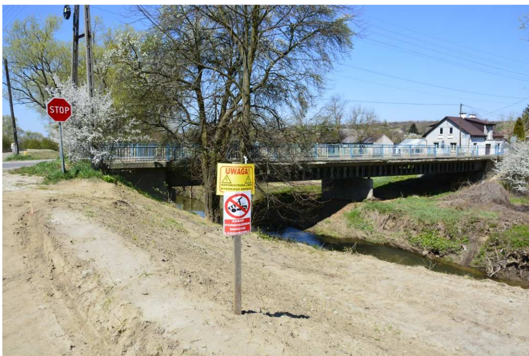
Fig. 16. Protection of hazardous sites – right bank of Koprzywianka river downstream of the bridge on the road no. 758 in Koprzywnica, status in the third decade of April 2021 (upstream view).
