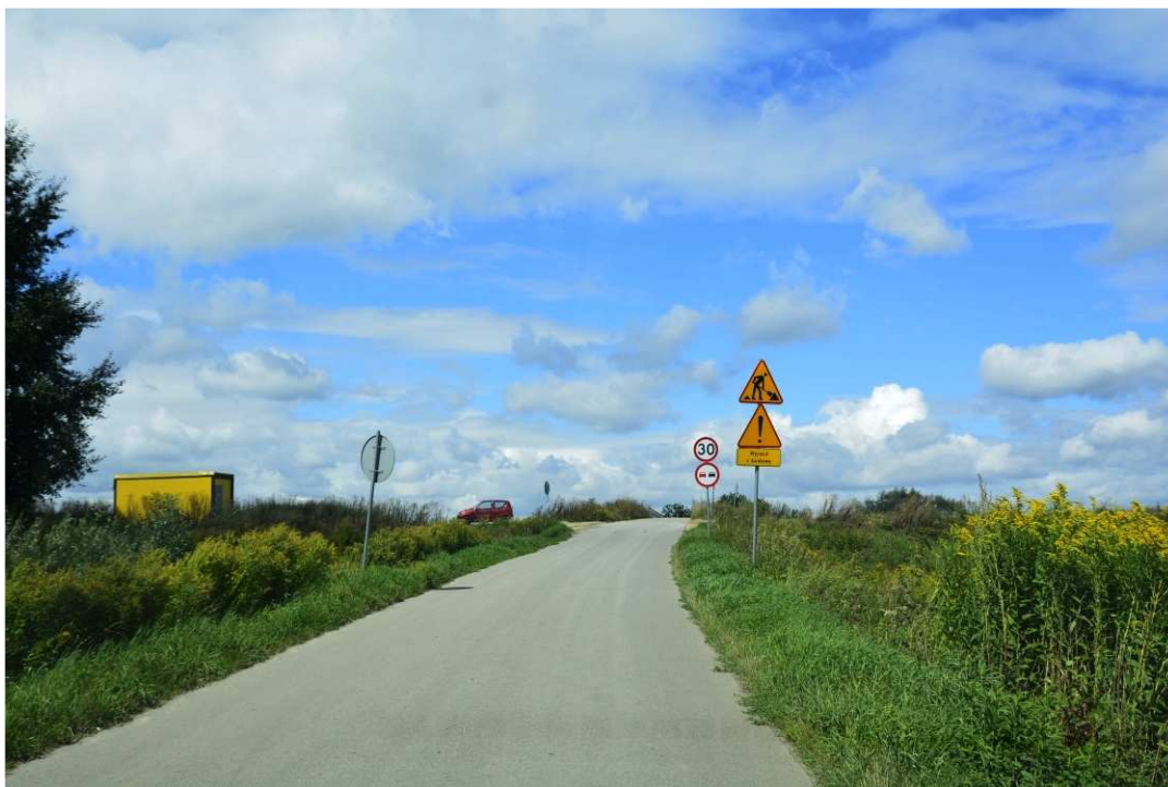
Fig. 13. Marking of public road near the exit from the construction site – right bank of Koprzywianka river at the bridge on the road Andruszkowice-Koćmierzów, status in the third decade of August 2020 (view towards the north-west).
