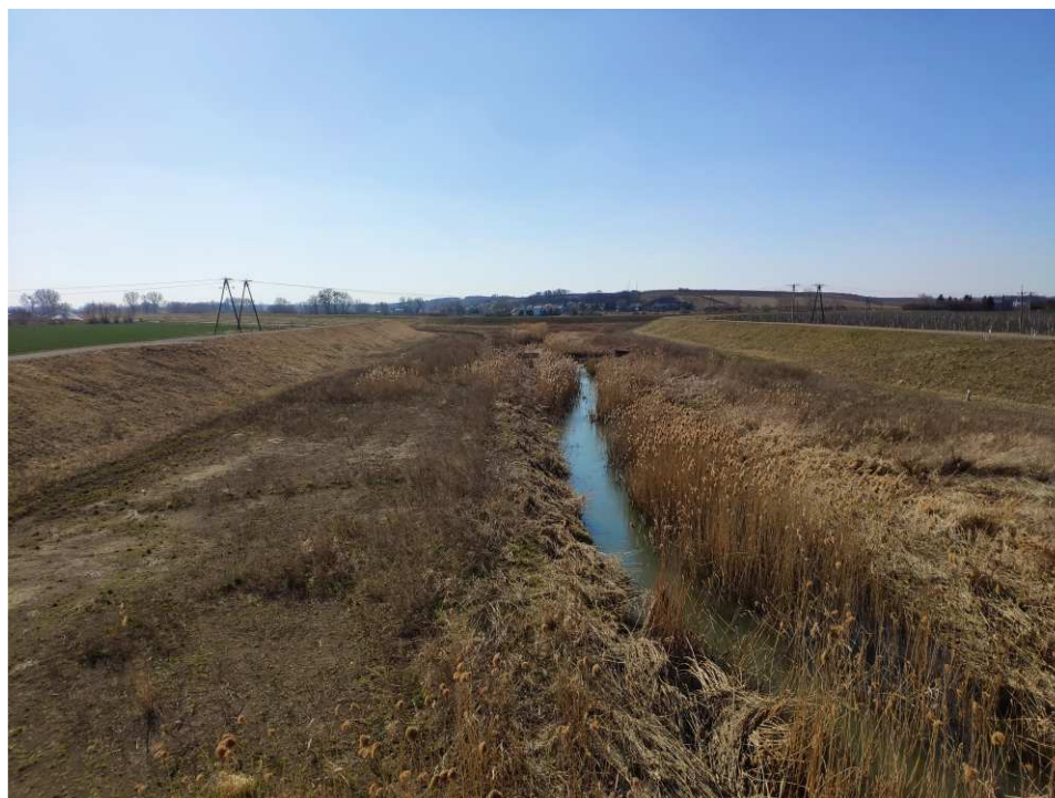
Fig. 52. Site condition in the last quarter of the works implementation period on Task 4 – banks of Koprzywianka river upstream of the bridge on the road Samborzec-Zajeziorko, status in the third decade of March 2022 (upstream view).
