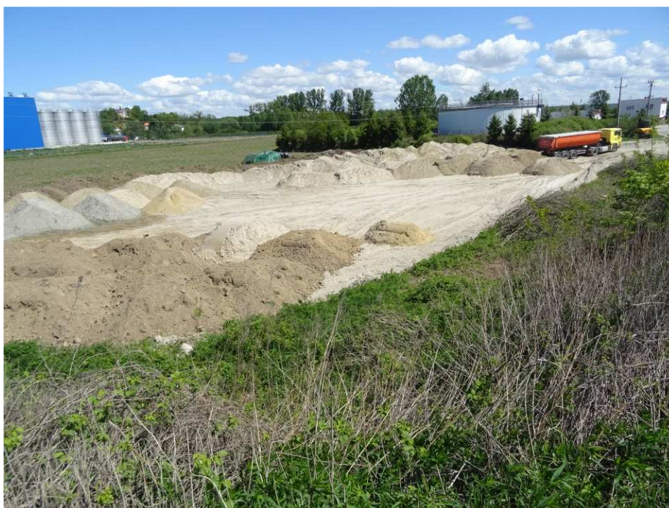
Fig. 10. Storage yard in the area beyond the left Koprzywianka embankment – left bank of Koprzywianka river downstream of the bridge on the road Samborzec-Zajeziorko, status in the second decade of May 2020 (downstream view).
