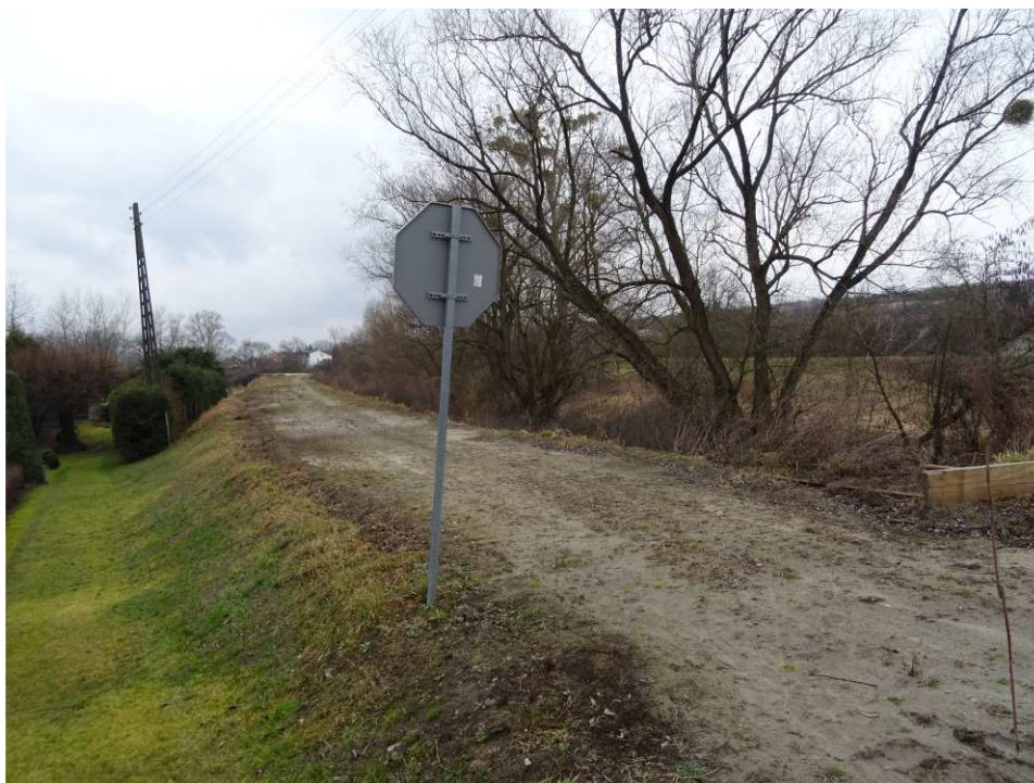
Fig. 8. Site condition in the first quarter of the works implementation period on Task 4 – right bank of Koprzywnianka river upstream of the bridge on the road no. 758 in Koprzywnica, status in the third decade of February 2020 (upstream view).
