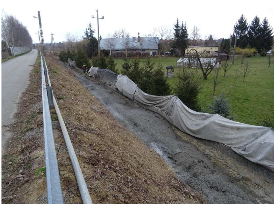
Fig. 19. Protection of trees and shrubs not intended to felling – band embankment within the artery of Mostowa Street, status in the third decade of March 2020 (view towards the north-east).
