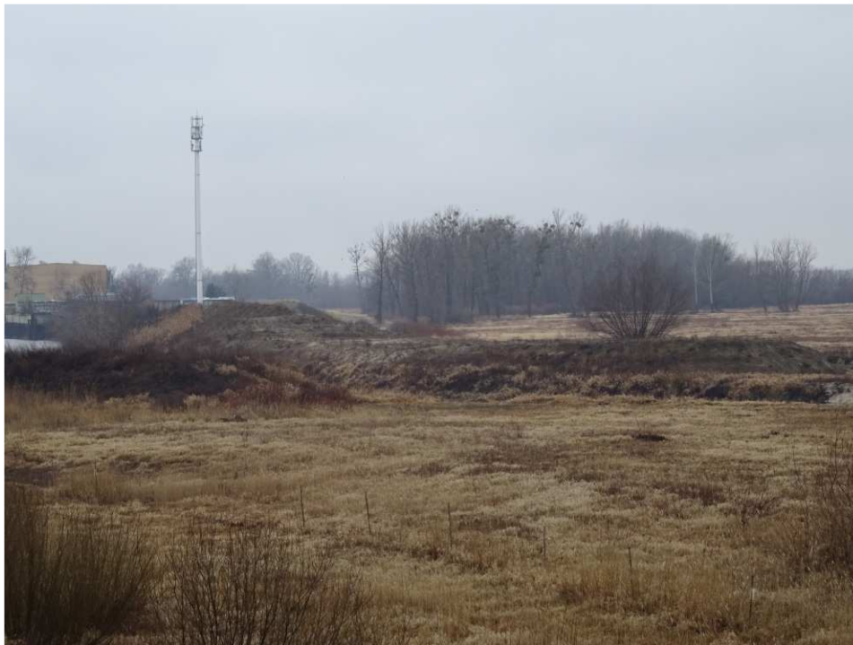
Fig. 1. Site condition in the first quarter of the works implementation period on Task 3 – planned flood gate on the port channel in Sandomierz, status in the third decade of February 2020 (view towards the west).
