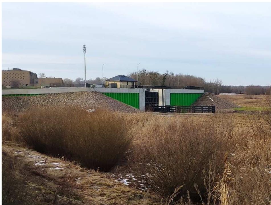
Fig. 49. Site condition in the last quarter of the works implementation period on Task 3 – flood gate on the port channel in Sandomierz, status in the third decade of December 2022 (view towards the west).
