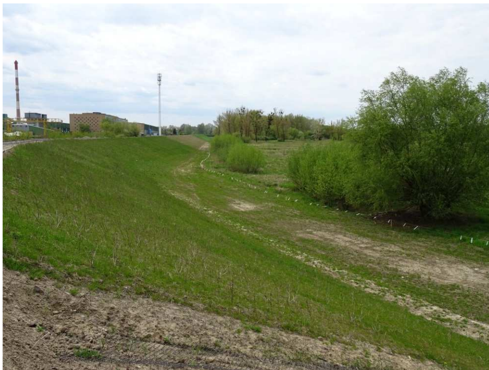
Fig. 40. Growth of grasses sown on the slope of the flood embankment – right-bank Vistula embankment along the bank of the port channel, status in the first decade of May 2022 (view towards the south-west).
