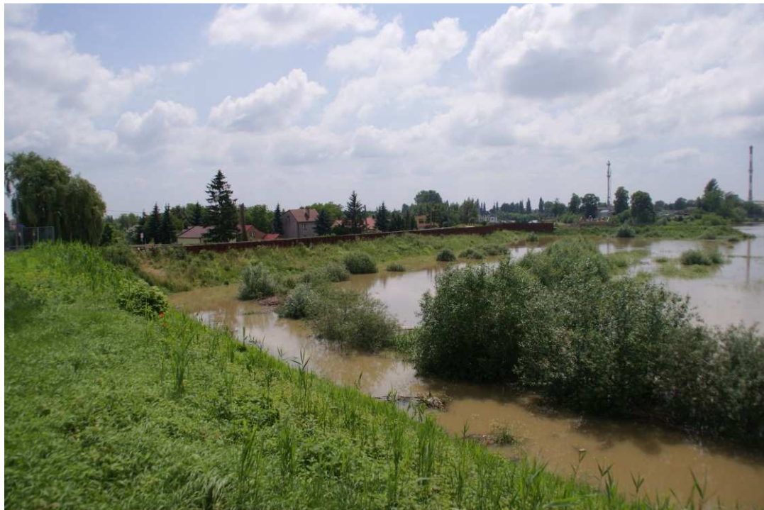
Fig. 41. Flooding from Vistula in the area of works – band embankment within the artery of Mostowa Street, status in the third decade of June 2020 (view towards the south-west).
