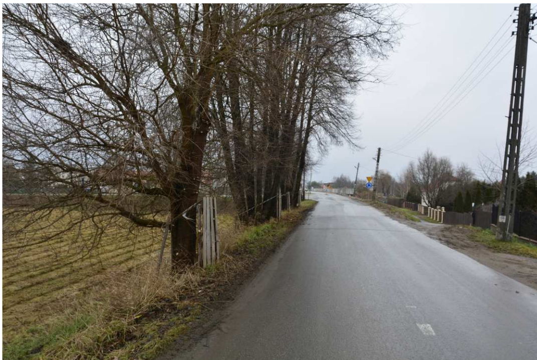
Fig. 20. Protection of trees and shrubs not intended to felling – band embankment within the artery of Zarzekowice Street, status in the second decade of December 2021 (view towards the north-east).
