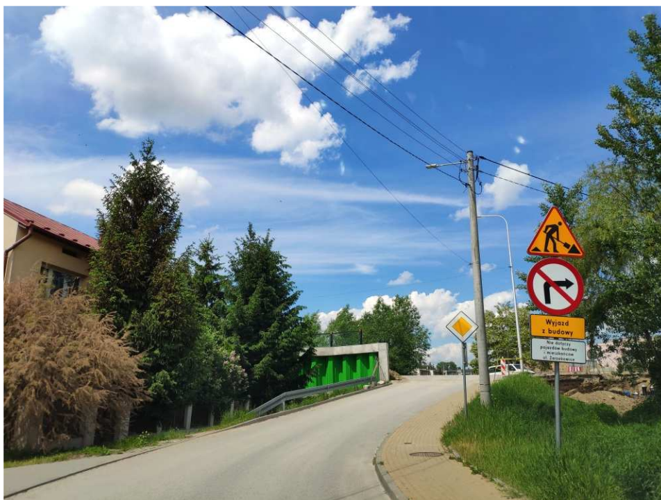
Fig. 16. Marking of public road near the exit from the construction site – band embankment within the artery of Zarzekowice Street, status in the third decade of May 2022 (view towards the south-west).
