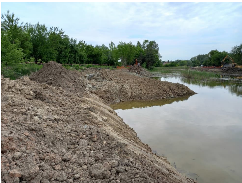
Fig. 45. Earthworks on the northern bank of the redeveloped reservoir on the Ditch 2, status in the third decade of May 2022 (view towards the east).
