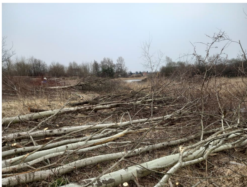
Fig. 14. Tree felling on the northern bank of the reservoir on the Ditch 2, status in the second half of March 2022 (view towards the east).
