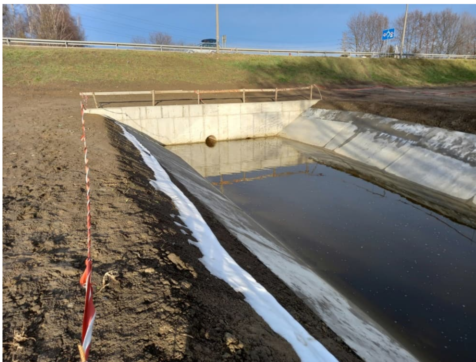
Fig. 21. Protection of hazardous sites on the construction area of embankment lock on the Ditch 2a within the embanked area of the Vistula River, status in the third decade of December 2022 (view towards the north).
