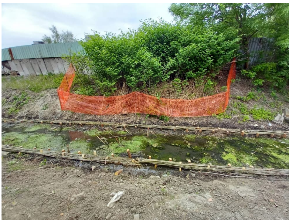
Fig. 26. Preventing the spread of foreign invasive plant species – fencing off knotweed site on the northern bank of the Ditch 2, status in the third decade of May 2022 (view towards the north).
