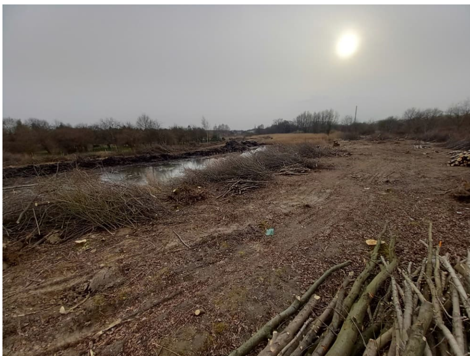
Fig. 10. Site condition in the first month of the works implementation period – redeveloped reservoir on the Ditch 2, western part, status in the third decade of March 2022 (view towards the west).
