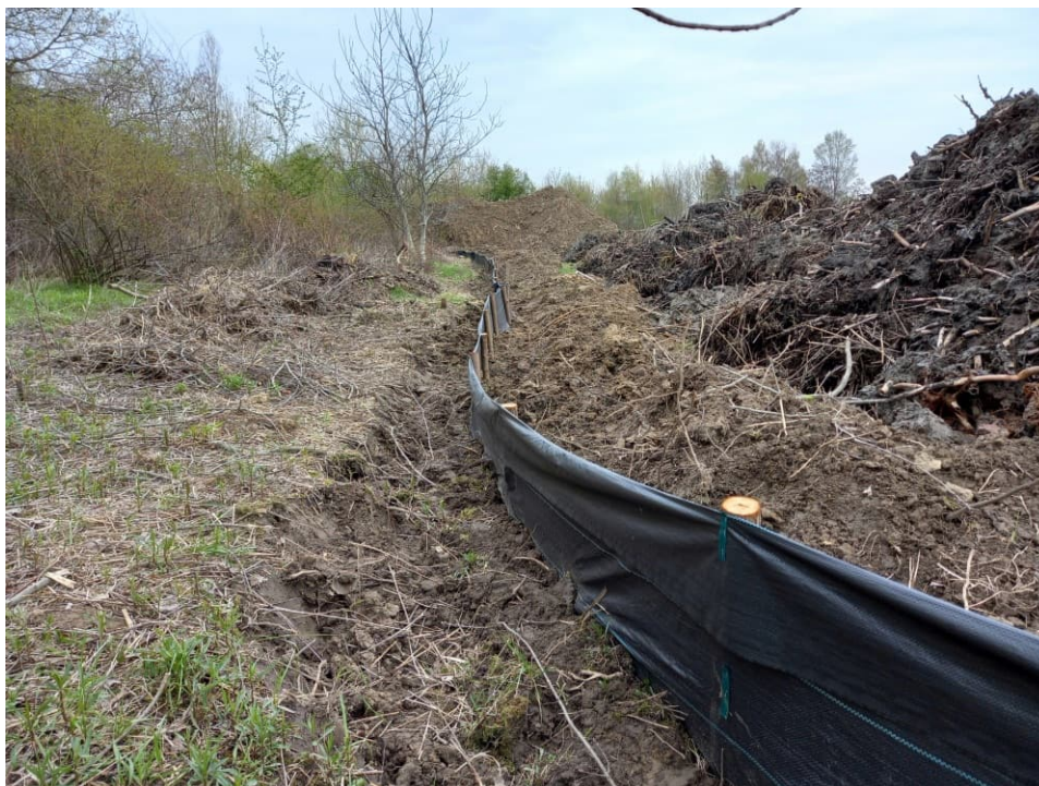
Fig. 30. Herpetological fence on the northern bank of the redeveloped reservoir on the Ditch 2, status in the third decade of April 2022 (view towards the east).
