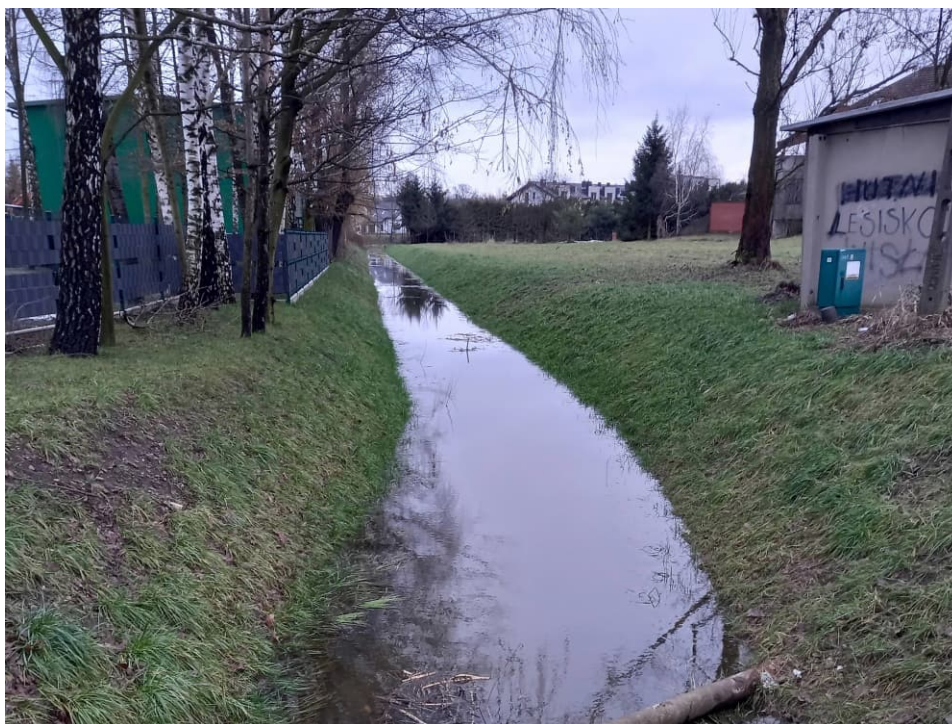
Fig. 55. Site condition in the last month of the works implementation period – redeveloped section of the Ditch 2 – downstream part, status in the third decade of January 2023 (view towards the east).
