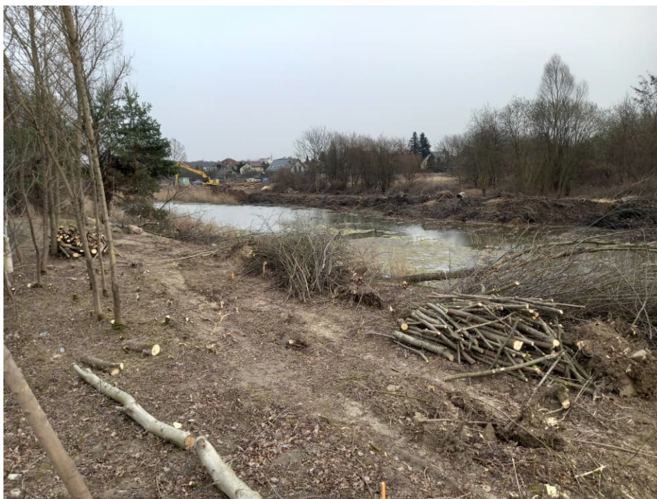
Fig. 9. Site condition in the first month of the works implementation period – redeveloped reservoir on the Ditch 2, eastern part, status in the third decade of March 2022 (view towards the east).
