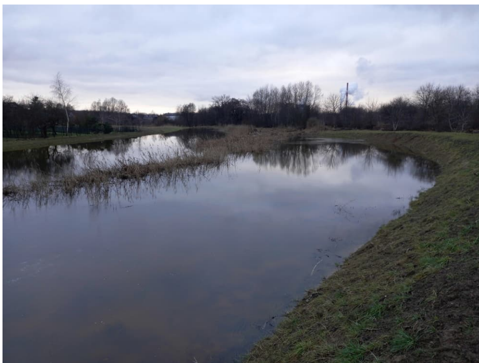
Fig. 58. Site condition in the last month of the works implementation period – redeveloped reservoir on the Ditch 2, western part, status in the third decade of January 2023 (view towards the west).
