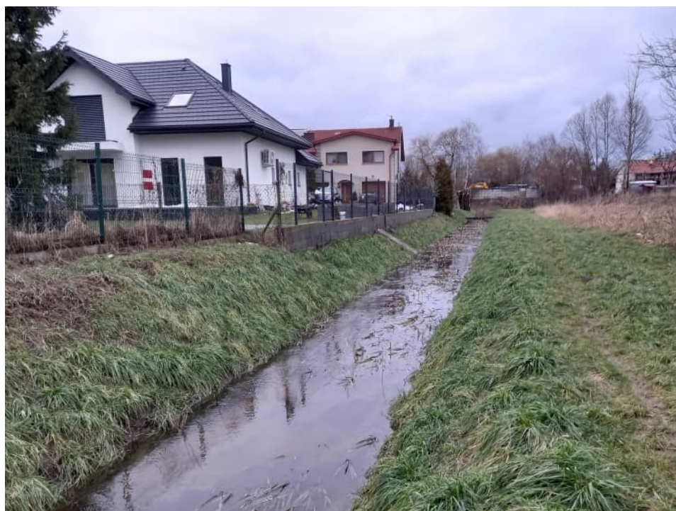
Fig. 54. Site condition in the last month of the works implementation period – redeveloped section of the Ditch 2a – upstream part, status in the third decade of January 2023 (view towards the north).
