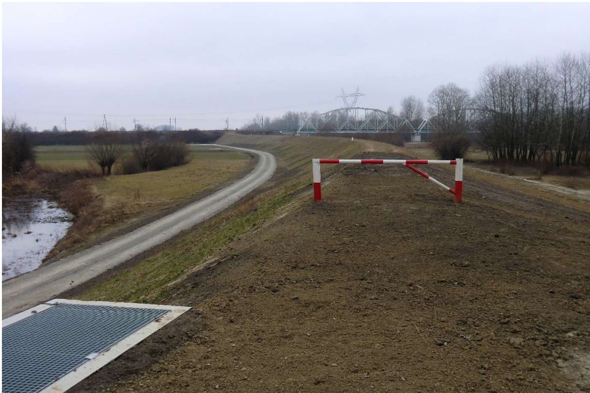
Photo no. 12. Extended embankment (Section III general view) (source: own materials of AECOM Polska Sp. z o.o.).
