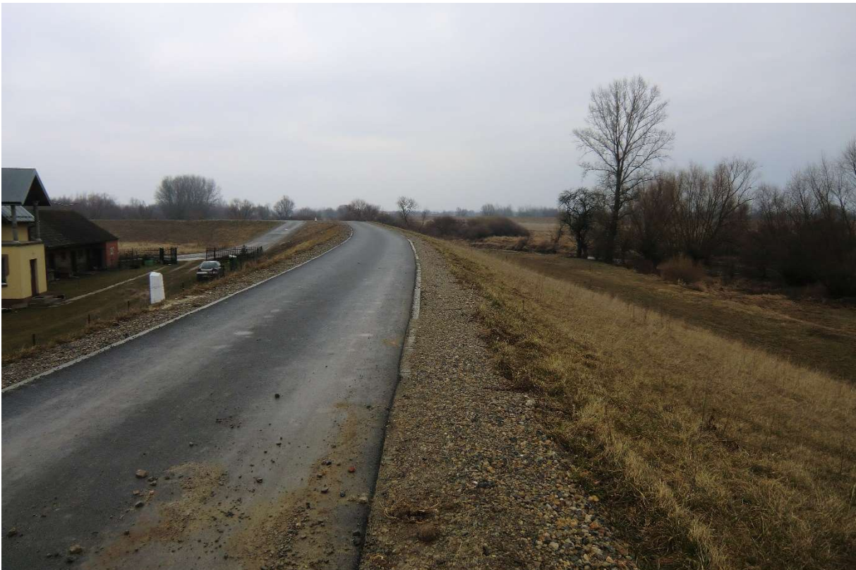
Photo no. 10. Extended embankment (Section III km 0+112) (source: own materials of AECOM Polska Sp. z o.o.).
