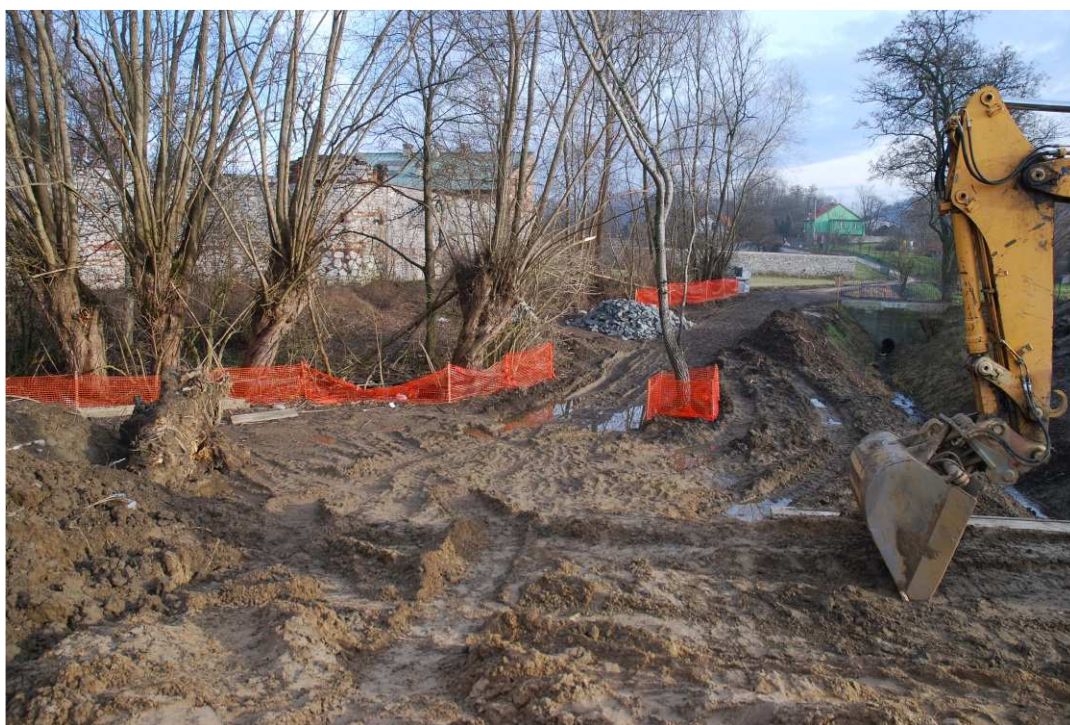
Fig. 19. Protection of trees and shrubs not intended to felling within Task 2 , status in the third decade of December 2020 (view towards the area beyond the embankment).
