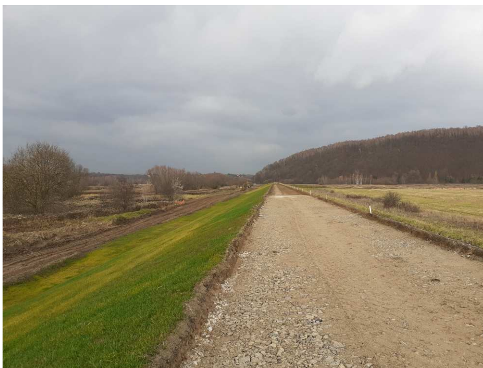
Fig. 39. Growth of grasses sown on the slope of the flood embankment within Task 1 , status in the third decade of November 2021 (downstream view).
