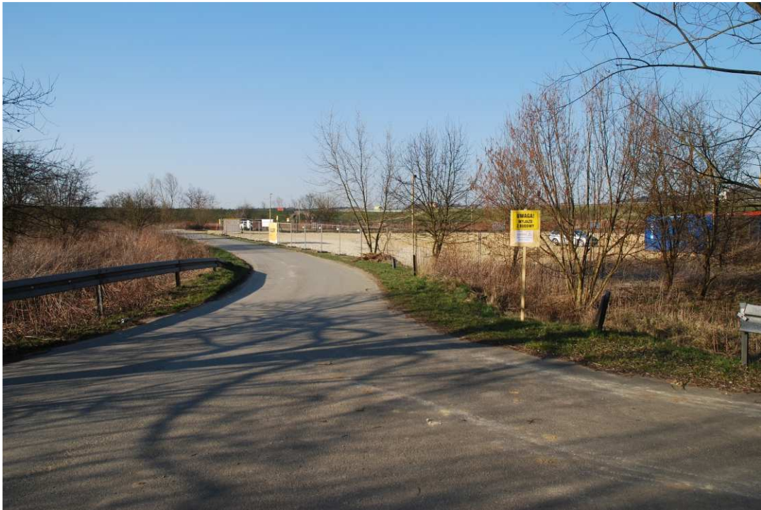
Fig. 11. Marking of the public road near the exit from the site facilities within Task 3 , status in the third decade of March 2020 (view towards the north).
