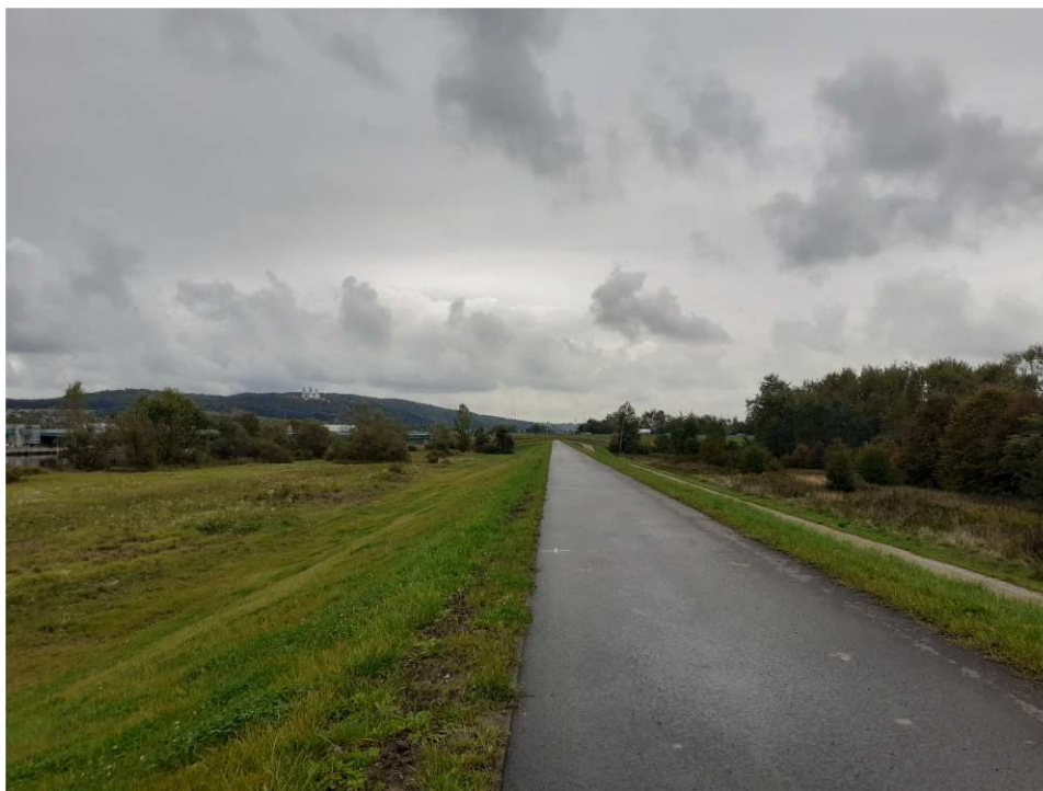
Fig. 46. Site condition in the last month of the works implementation period – the right Vistula embankment within Task 3 , status in the third decade of September 2022 (downstream view).
