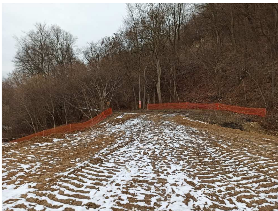
Fig. 18. Protection of trees and shrubs not intended to felling within Task 1 , status in the third decade of January 2021 (downstream view).
