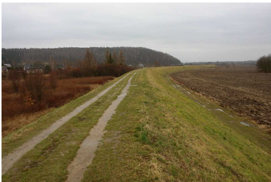
Fig. 3. Site condition in the first month of the works implementation period – the right Vistula embankment within Task 2 , status in the third decade of February 2020 (upstream view).
