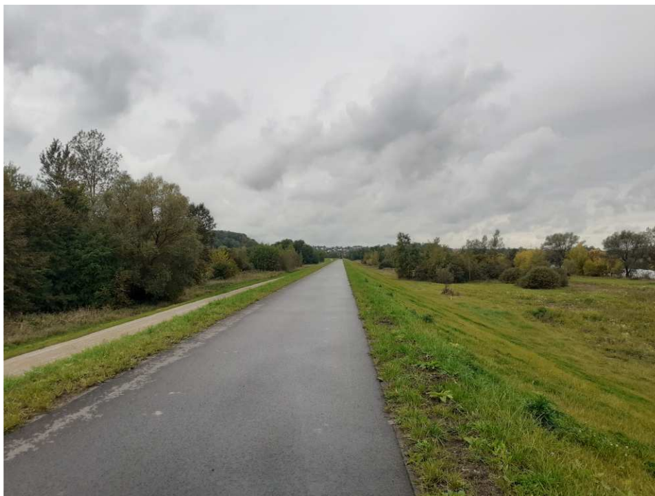
Fig. 45. Site condition in the last month of the works implementation period – the right Vistula embankment within Task 3 , status in the third decade of September 2022 (upstream view).
