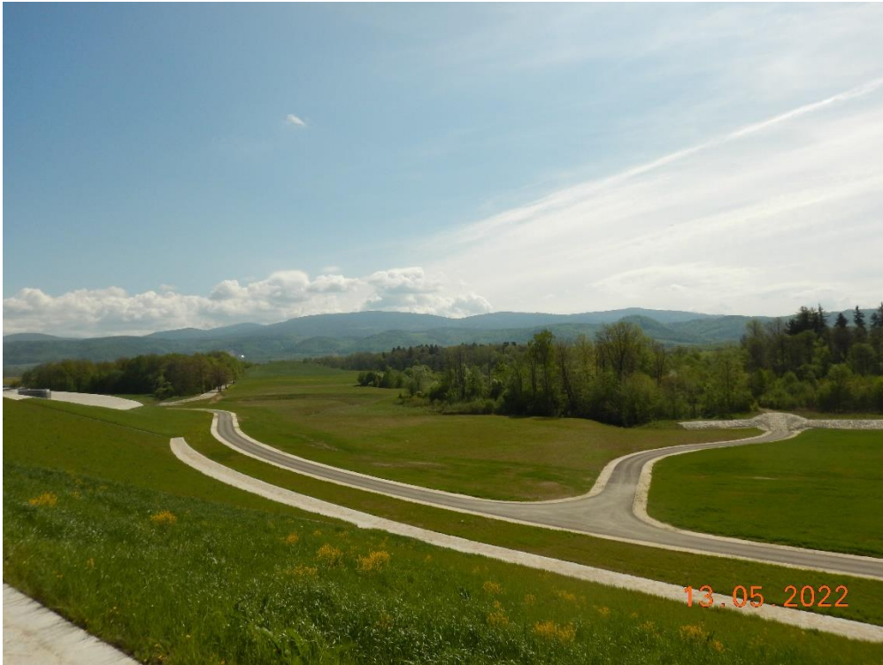
Photo.7. Reservoir basin - visible growth of mixture of grasses (Defects Notification Period).
