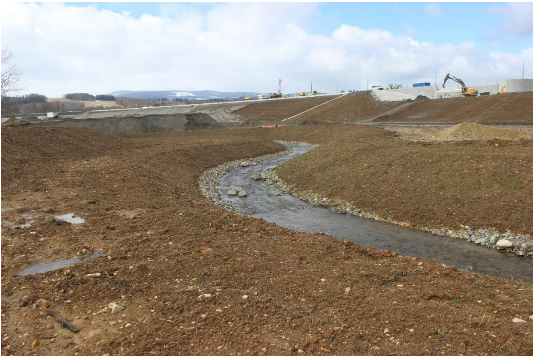
Photo.2. New stream bed of Nowinka, slopes of the stream have been topsoiled and seeded with a mixture of grasses - Contract implementation stage.
