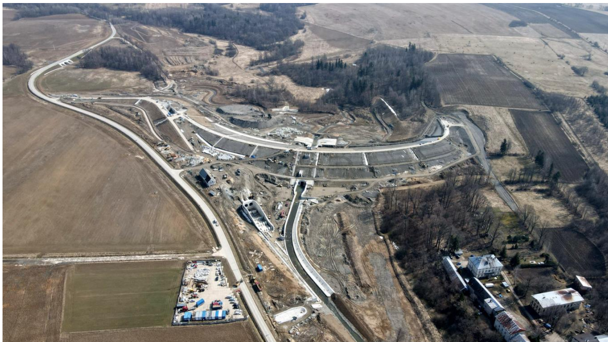
Photo.10. Works execution for 2A.1/2 Contract – March 2021.
