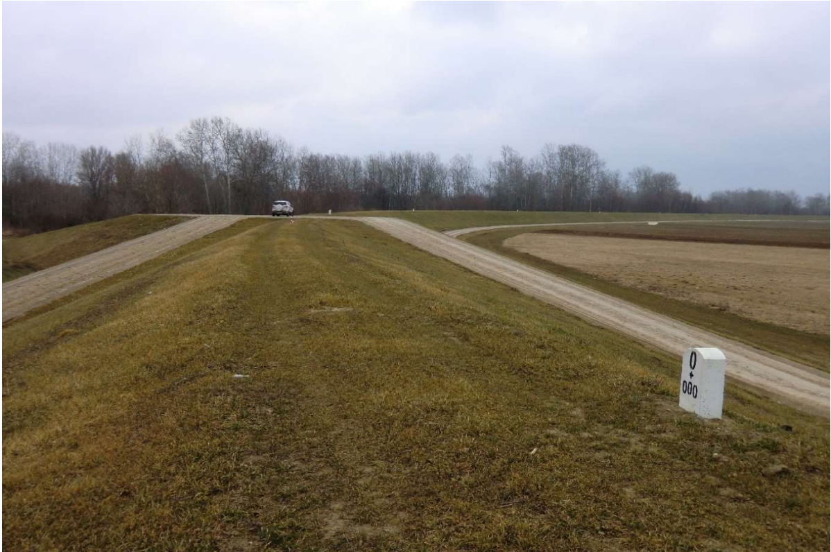
Photo no. 1. Completed embankment redevelopment (San III km 0.4 – general view) (source: own materials of AECOM Polska Sp. z o.o.).
