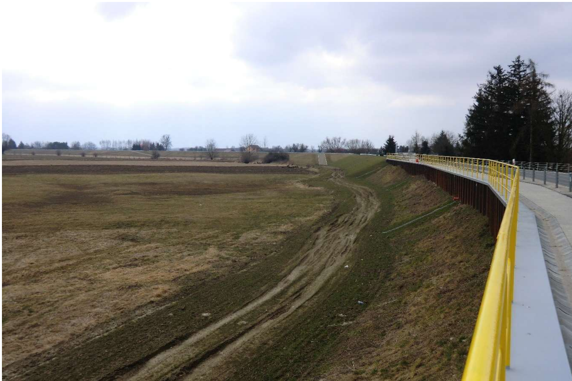
Photo no. 3. Completed embankment redevelopment (San III km 2.955 – raising of embankment crest datum by a retaining wall with a top-plate and a protective barrier) (source: own materials of AECOM Polska Sp. z o.o.).
