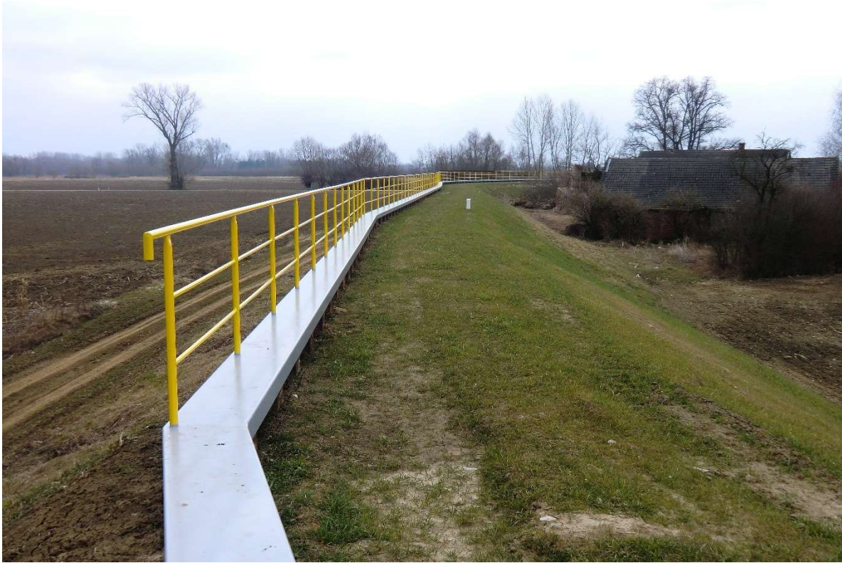
Photo no. 3. Completed embankment redevelopment (San III km 2.955 – raising of embankment crest datum by a retaining wall with a top-plate and a protective barrier) (source: own materials of AECOM Polska Sp. z o.o.).
