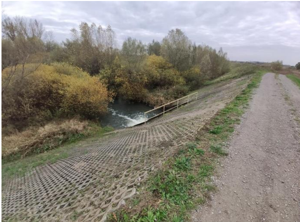
Photo no. 8: Discharge of water from the pumping station of PGW WP to the embanked area.
