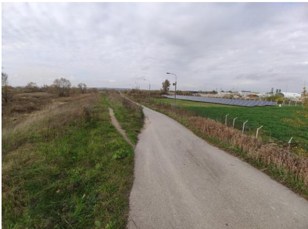
Photo no. 10: Asphalt exit road from the embankment, photovoltaic power plant in the background.
