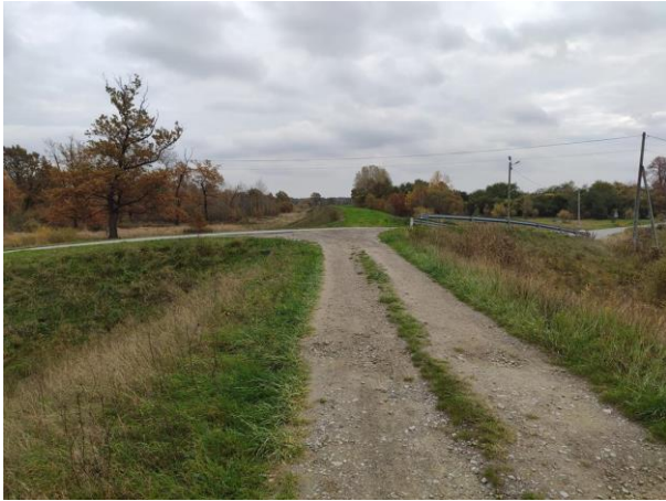
Photo no. 15: End of the investment – road Orliśka – Gorzyce.
