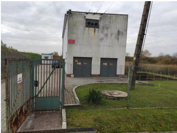
Photo no. 7: Pumping station of PGW WP, Strug water-course.
