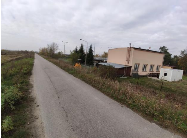
Photo no. 6: Treatment plant's buildings.
