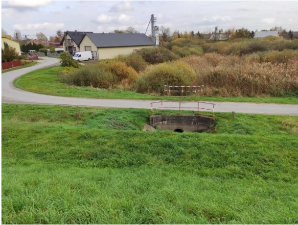
Photo no. 18: Culvert underneath Podwale Street.
