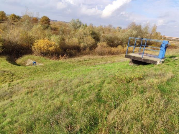
Photo no. 12: Culvert spanning through the embankment, valve.
