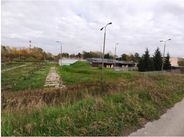
Photo no. 9: Objects of waste treatment plant.
