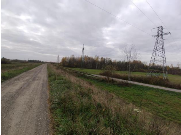
Photo no. 3: HV line spanning over the investment site.
