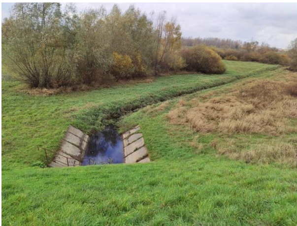
Photo no. 19: Discharge from the culvert on the embanked area's side (Podwale Street).
