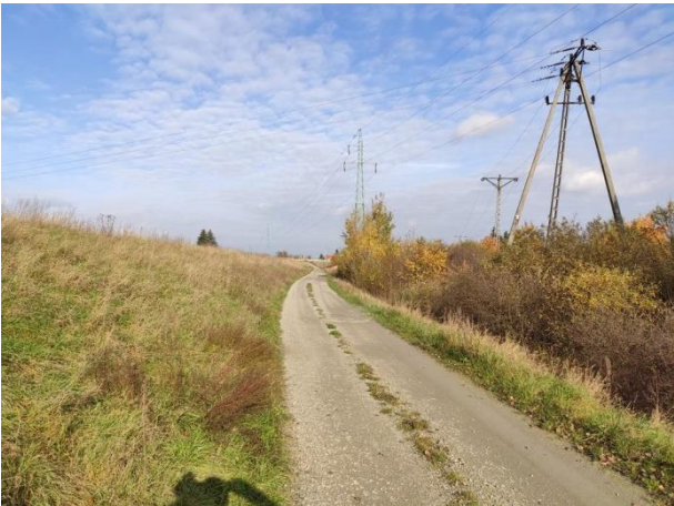
Photo no. 14: Embankment, road, HV and MV posts to be redeveloped.
