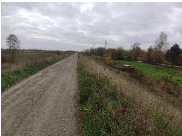
Photo no. 2: Foundations to be removed.
