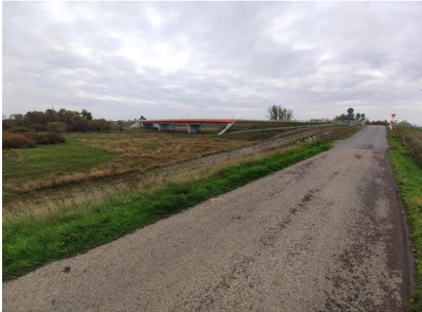
Photo no. 6: View on the bridge over the River Łęg , DK 77 (Sandomierska Street).
