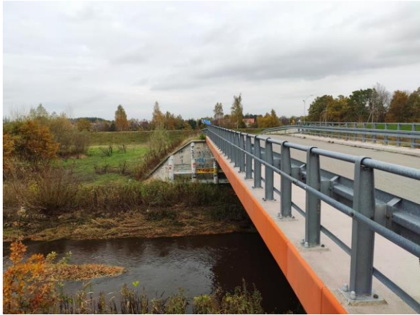
Photo no. 1: Bridge over the River Łęg, road Orlińska – Gorzyce.
