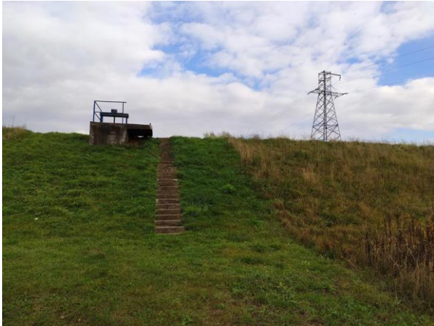
Photo no. 24: Culvert running through the embankment, valve, HV line.
