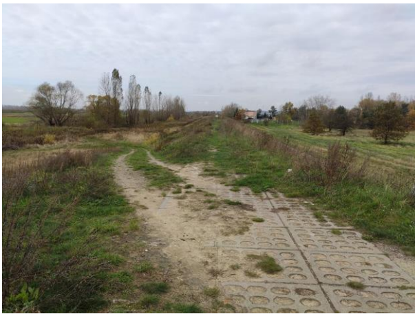
Photo no. 4: Paving of the passage crossing the embankment.
