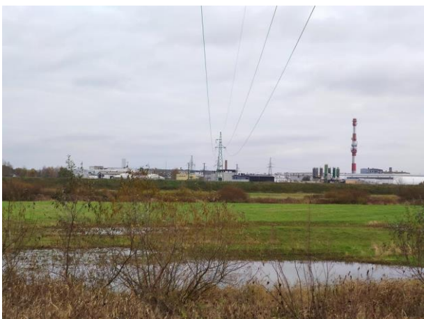
Photo no. 11: View on the embanked area River Łęg, industrial land in the background.
