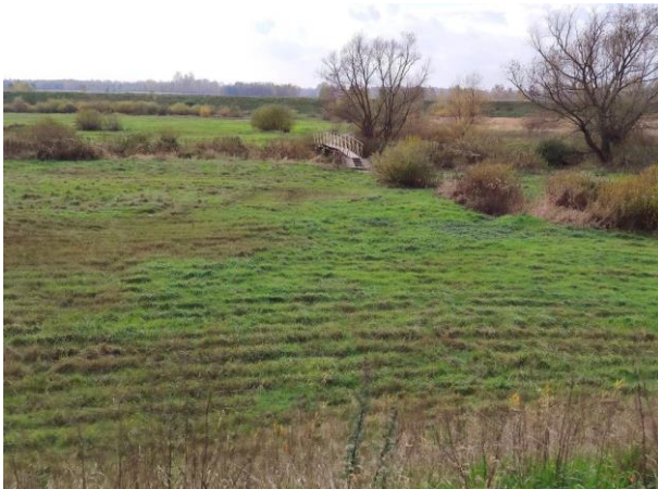
Photo no. 11: View from the right embankment on the footbridge.
