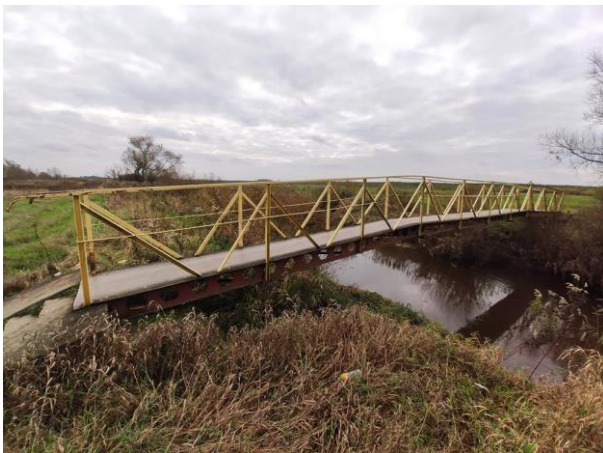
Photo no. 13: Footbridge over the River Łęg.
