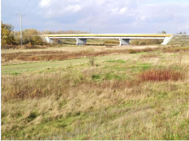
Photo no. 15: View from the right embankment on the bridge at DK 77, MV line.
