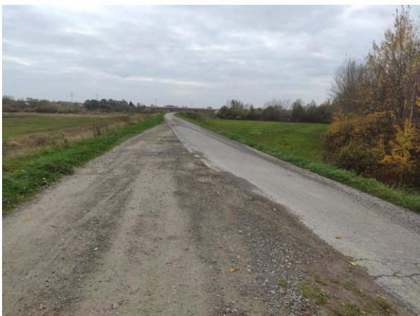
Photo no. 4: Crossing between the dirt road and the asphalt road – running on the top of embankment.
