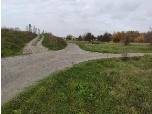
Photo no. 3: Crossing of roads with an access road onto the embankment, gas reduction station in the background.
