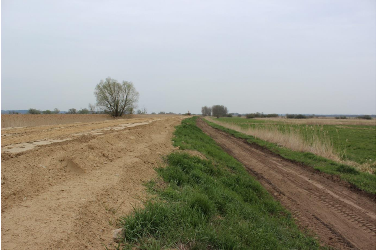
April 2021, Marwice - Krajnik, raising the embankment crown
