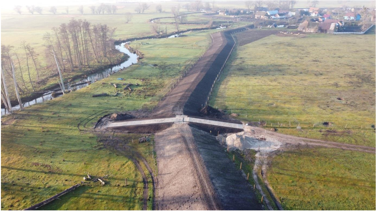
December 2020, Chlevice, flood embankment prepared for sowing grasses
