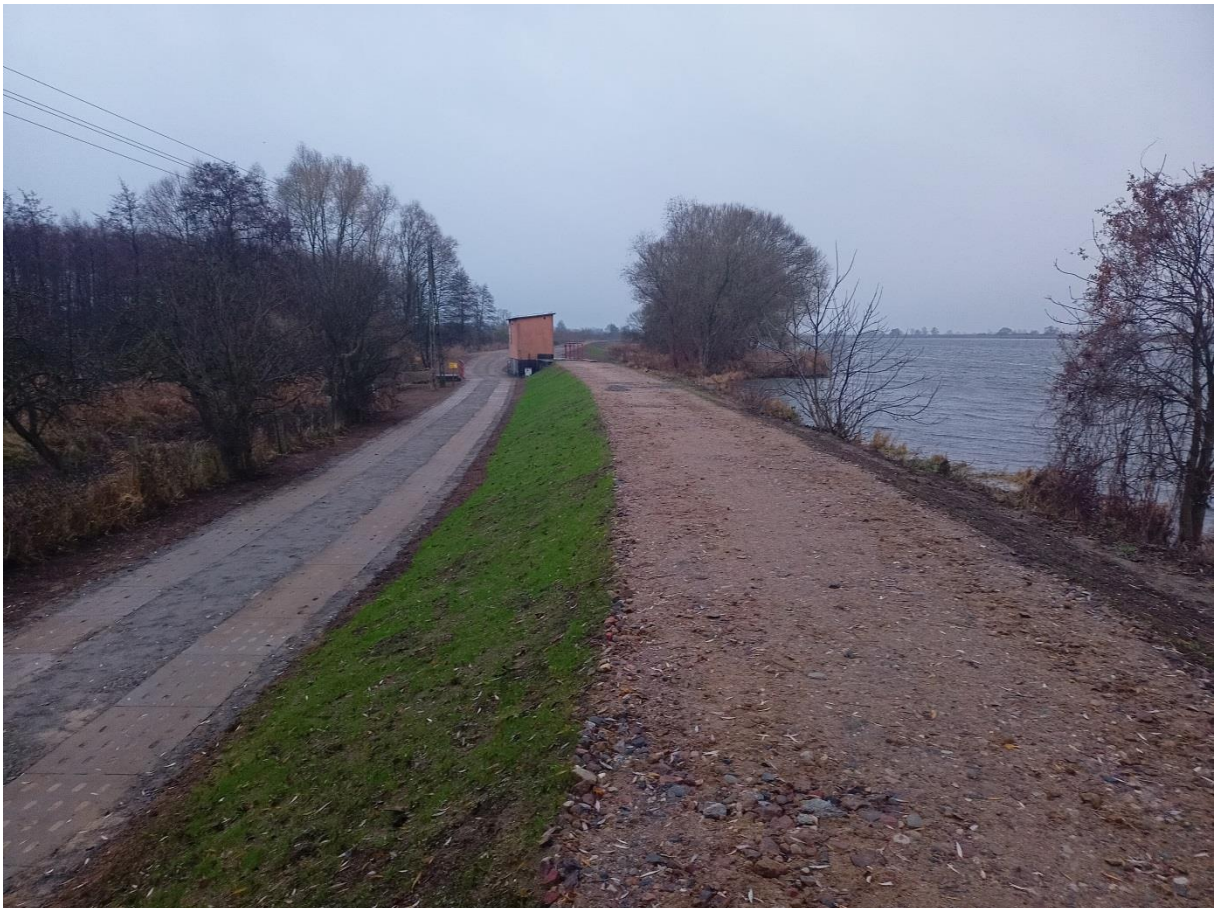
October 2021, Gryfino-Mniszki, completed embankment section
