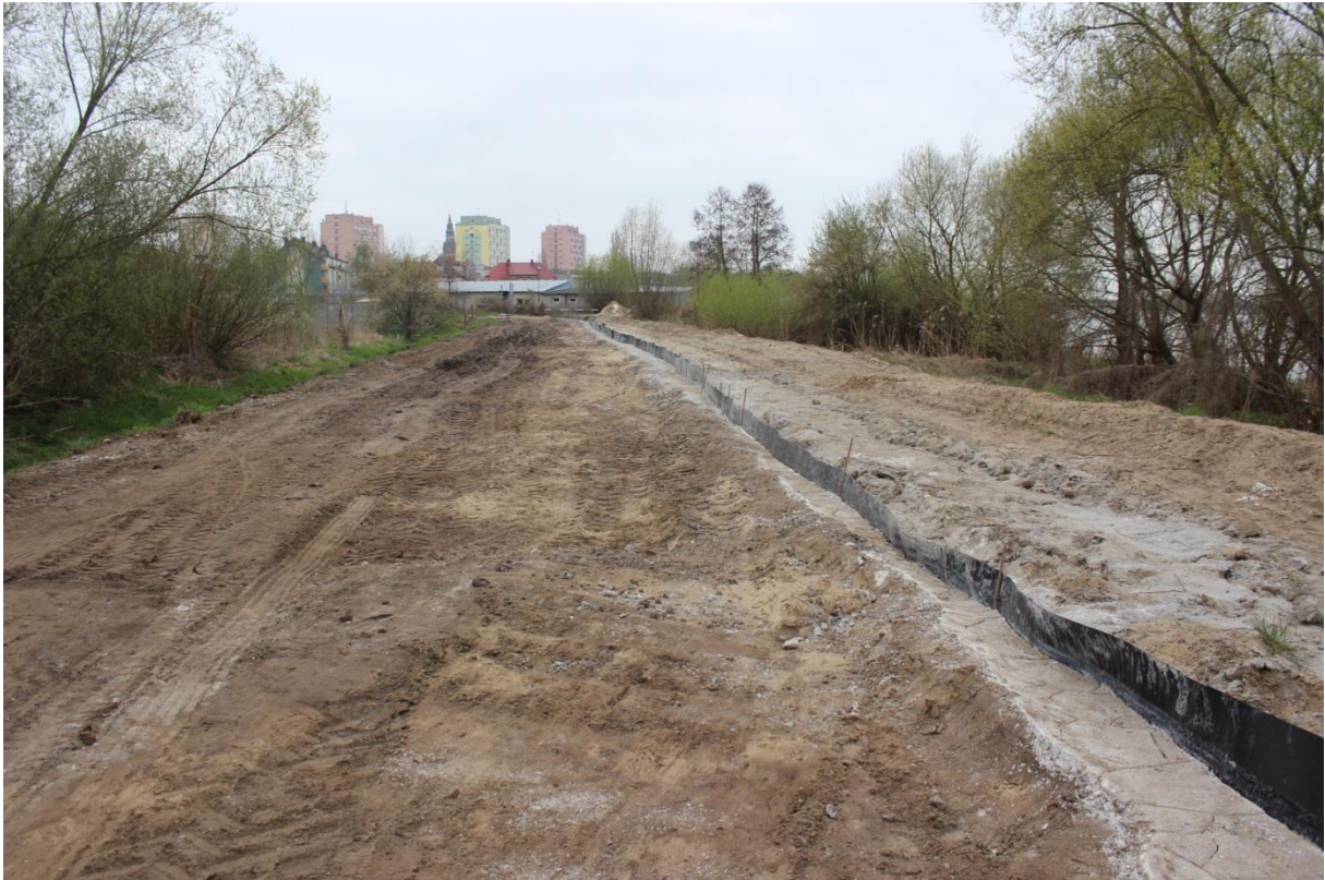
April 2021, Gryfino-Mniszki, constructed cut-off wall
