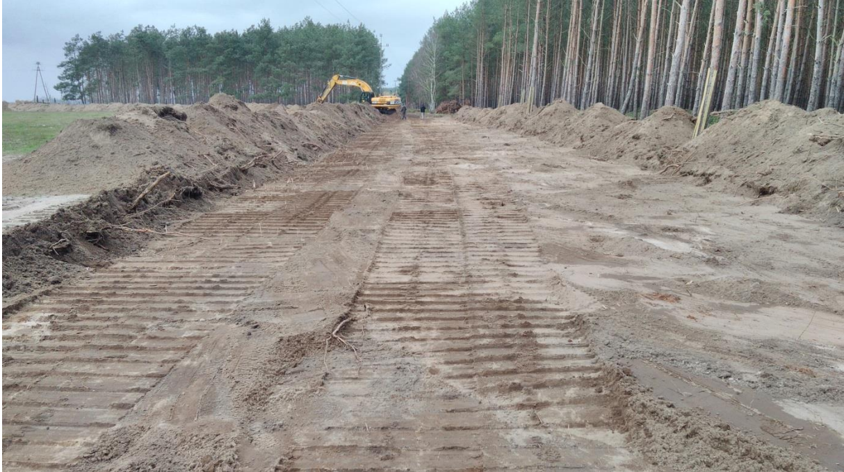
November 2017, Chlewice, removal of humus prior to the commencement of works
