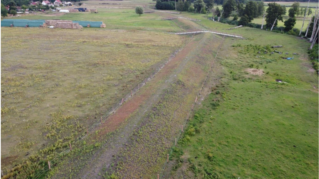
August 2021, Chlewice, greening of embankments
