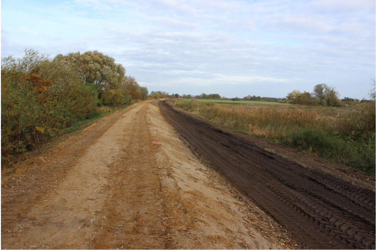
October 2021, Gryfino-Mniszki, embankment structure prepared for topsoiling
