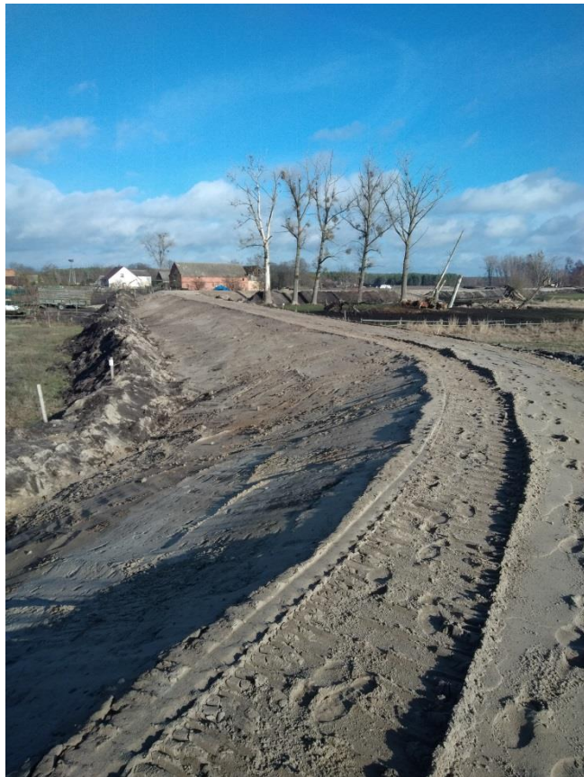
November 2017, Chlewice, removal of humus prior to the commencement of works
