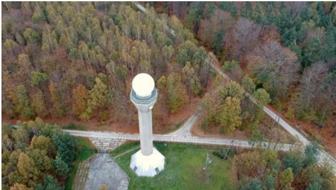
Photography 7 Location of the radar tower in Ramża - general view
