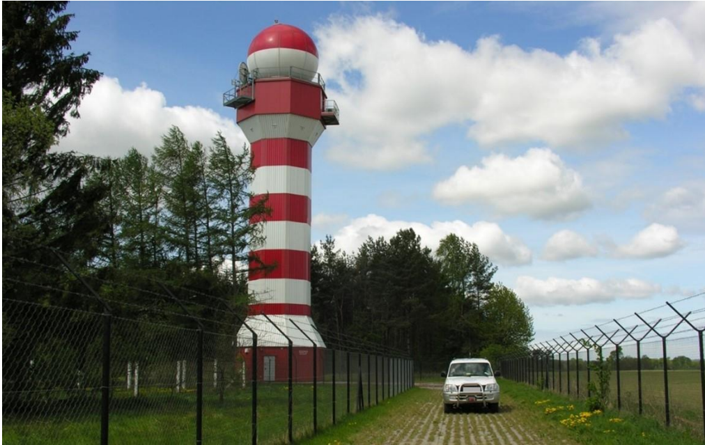
Photography 4 Location of the radar tower in Świdwin - general view
