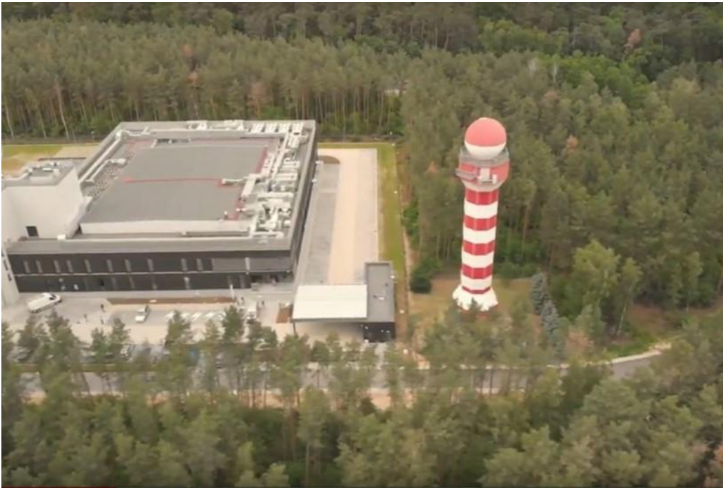
Photography 6 Location of the radar tower in Poznań - general view
