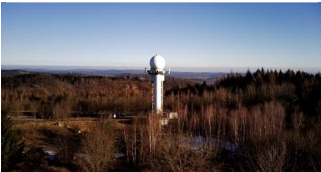
Photography 5 Location of the radar tower in Pastewnik - general view
