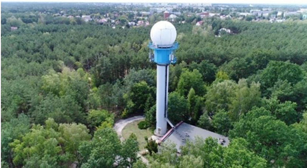
Photography 1 Location of the radar tower - general view
