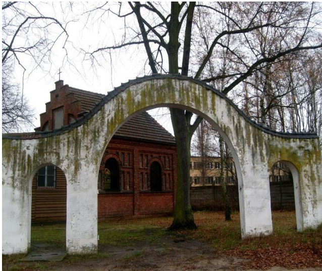
Fig. 2 The cemetery chapel from 1892 at Chocimska street; source: encyklopedia.szczecin.pl
