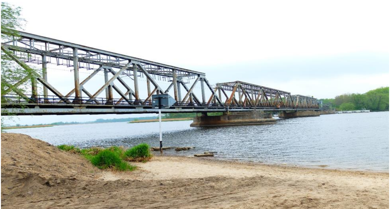
Photo 1: The existing railway bridge
