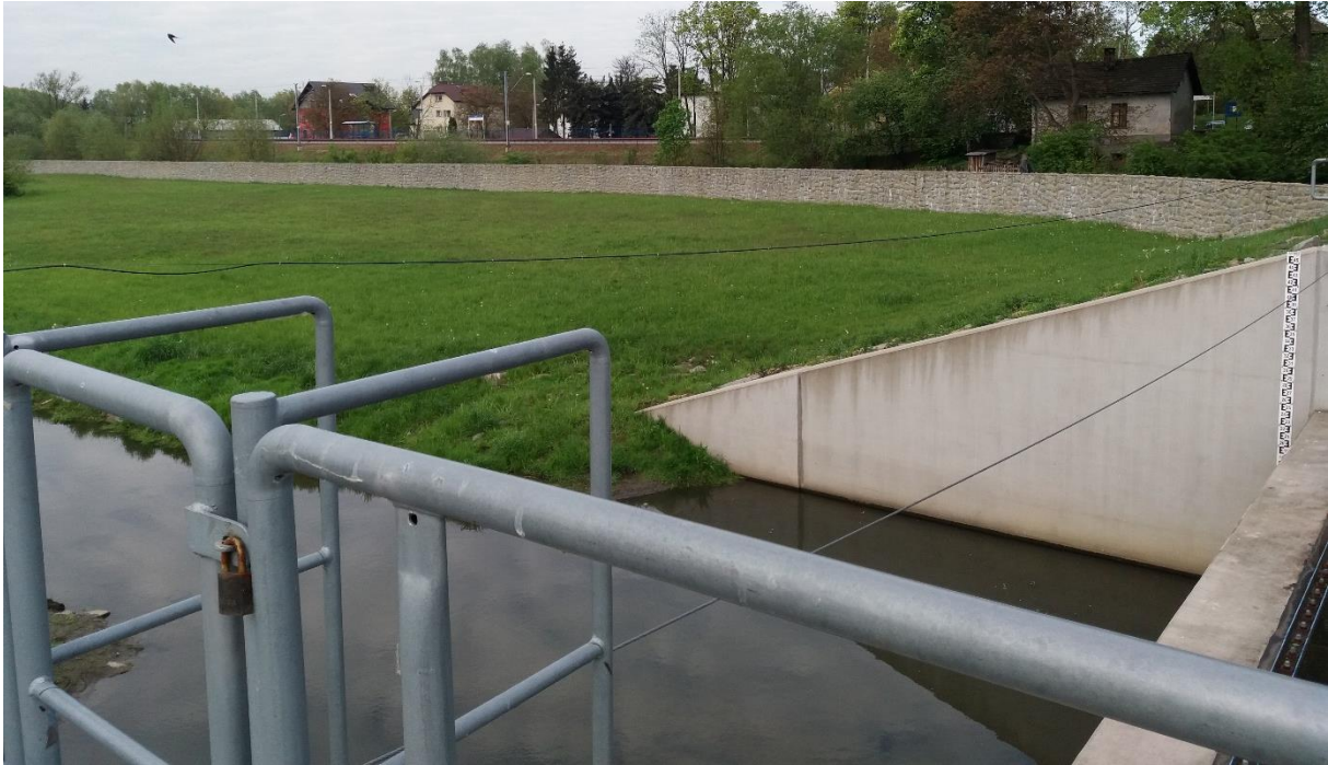
Photo 3: Example of maintenance of the Bieżańów reservoir
