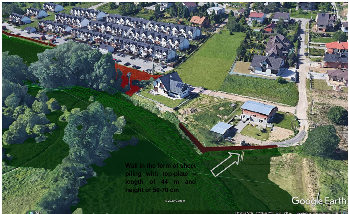
Figure 9. Planned retaining wall in the back water effect area on the right bank of the reservoir
