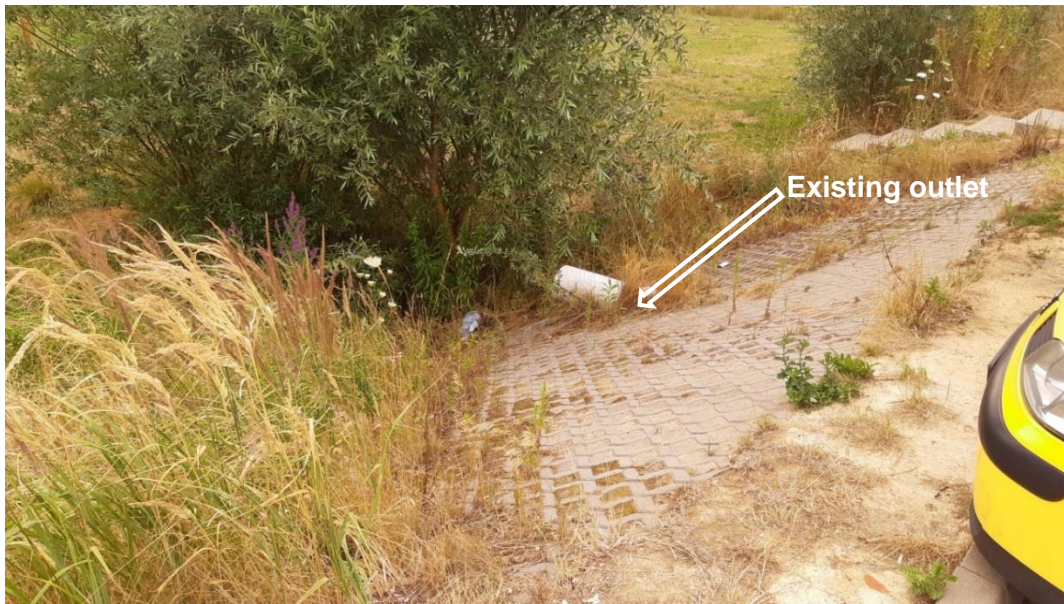
Photo 4: Existing rainwater outlet from the housing estate to the Malinówka stream's area near the river (the outlet will be rebuilt and the capacity of the rainwater drainage system increased).
