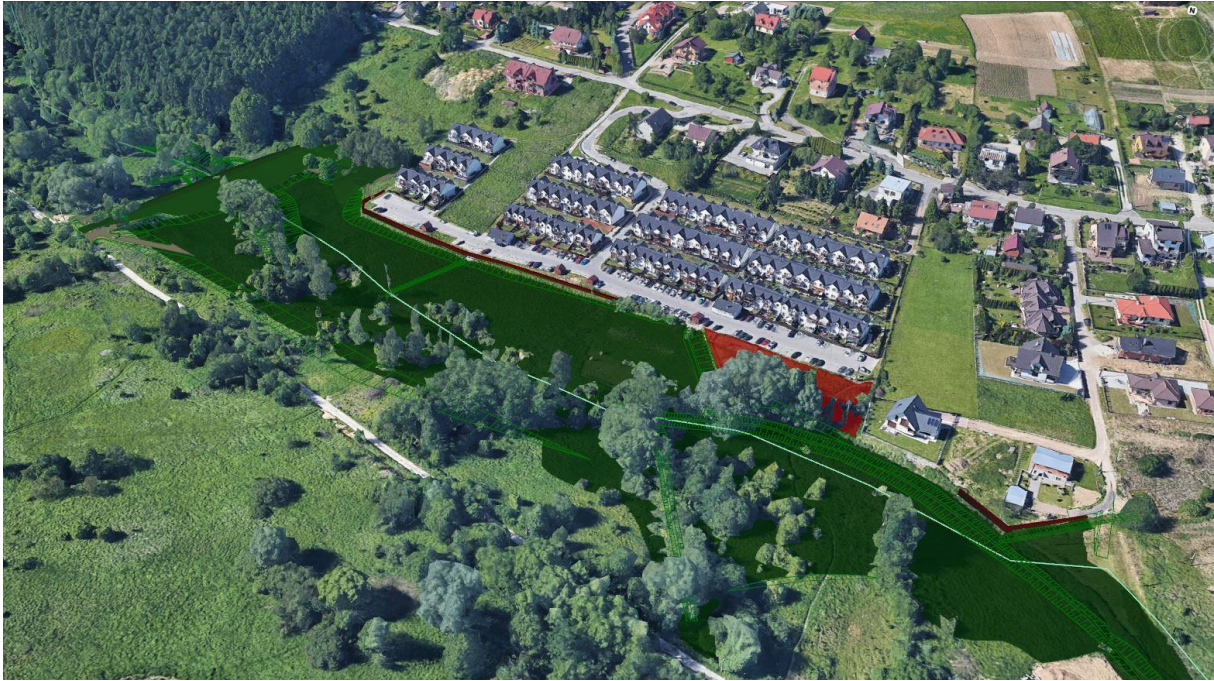
Figure 5. Planned status - the Secesja estate and the area where the bowl of Malinówka 3 reservoir will be implemented
