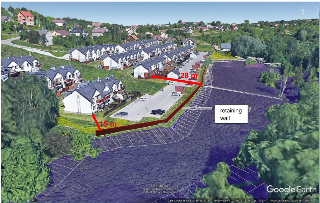
Figure 3. Planned status - the Secesja estate and the area where the bowl of Malinówka 3 reservoir will be implemented
