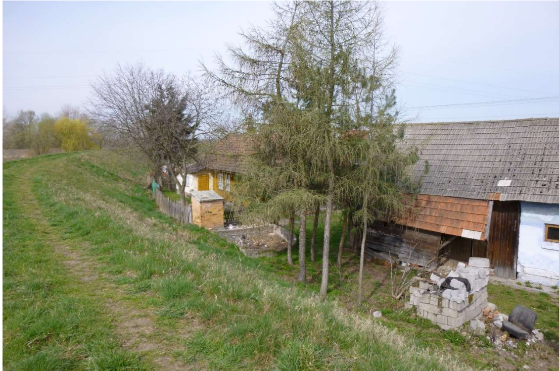
Photo no. 4 Right embankment 2+956 – 3+120 - the area beyond the embankment, buildings about 2.0 m from the embankment.
