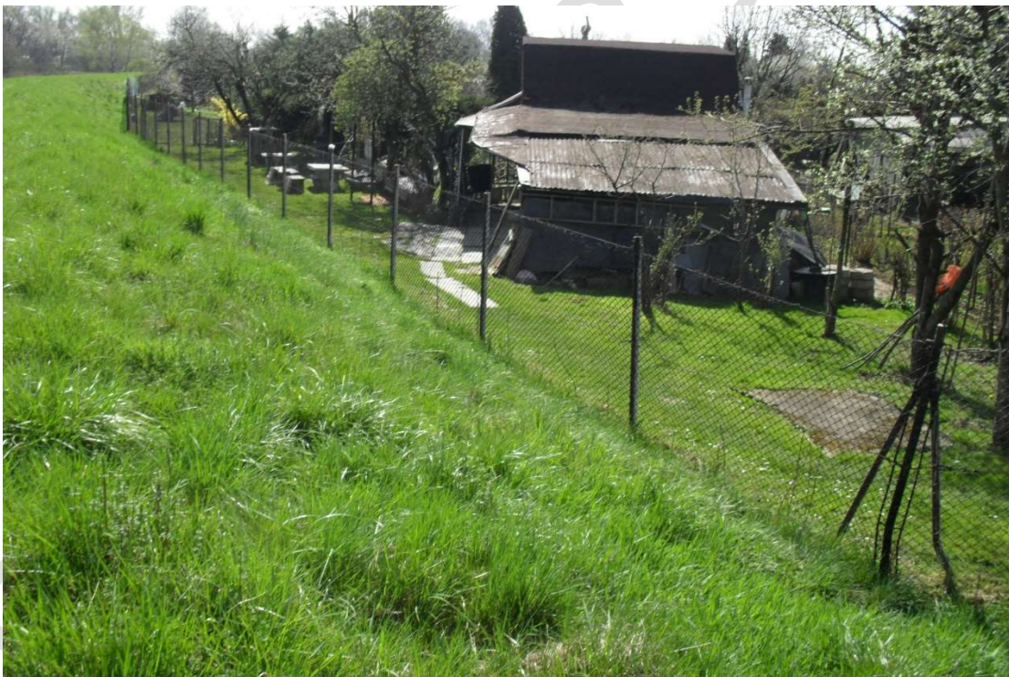
Photo no. 10 Left embankment - embanked area of the Family Allotment Gardens.
