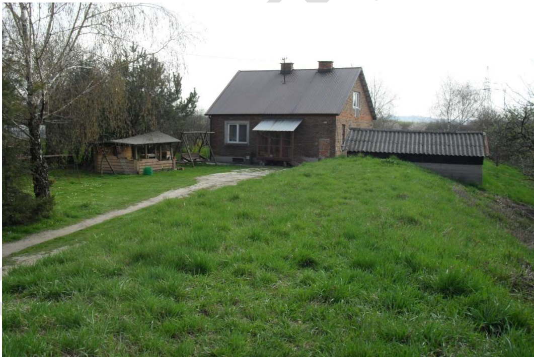
Photo no. 5 Right embankment 3+145 – 4+534 - residential building belonging to the Tarnów Municipality within the embankment crest, foreseen for demolition (currently uninhabited vacancy).
