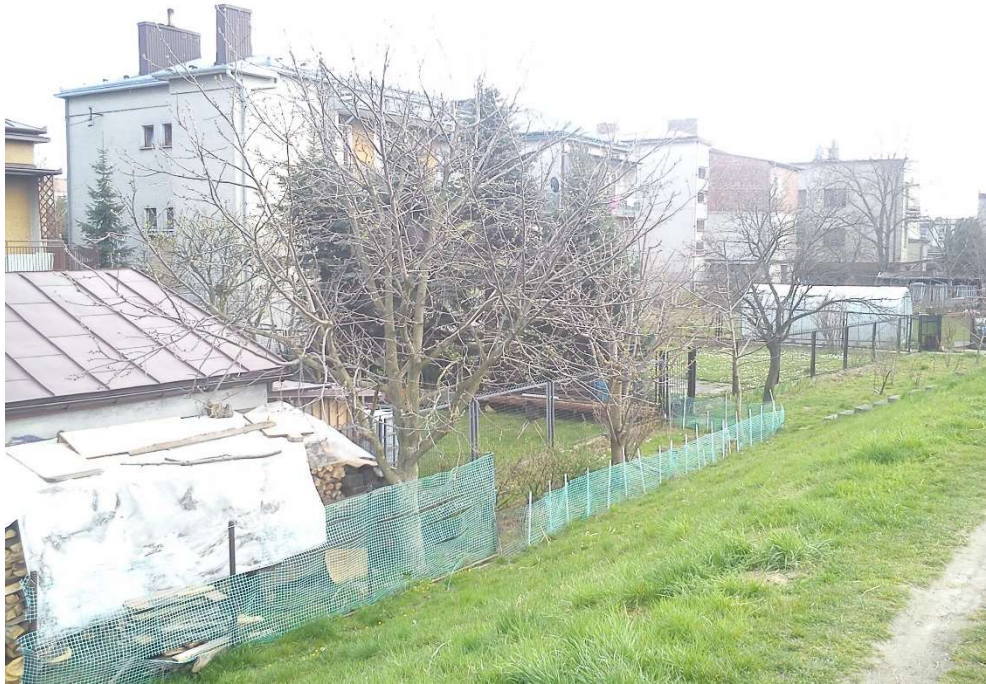
Photo no. 6 Right embankment 5+260 – 5+860 - outbuilding with a fence by the embankment (to be demolished).
