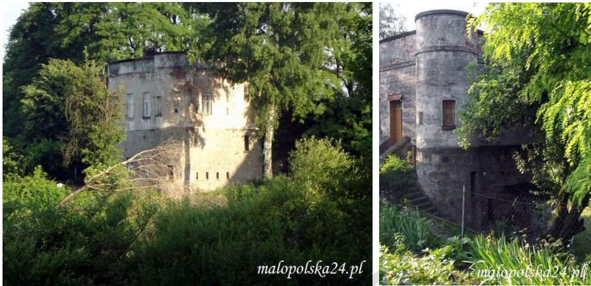
Photos no. 8 and 9. Railway gatehouse (at Kassali Street) at the railway bridge spanning the River Biala
