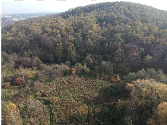
Photo no. 6: Works Contract 3A.2/2, Malinówka 2– investment implementation site – Source: own materials
