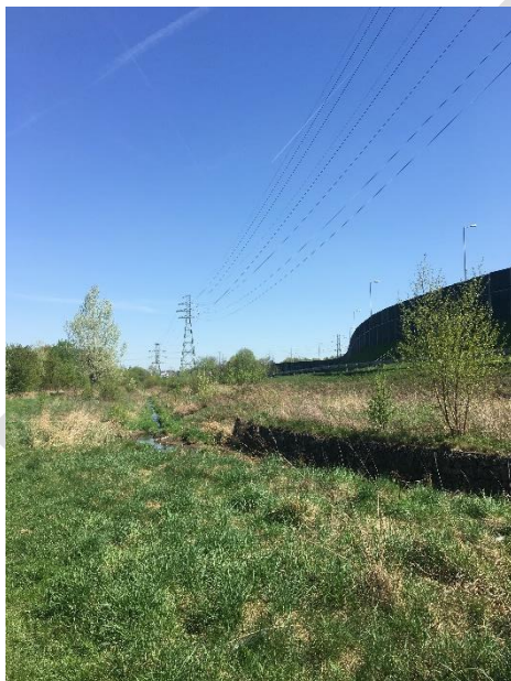
Photo no. 2: Works Contract 3A.2/1, Malinówka 1– investment implementation site – Source: own materials
