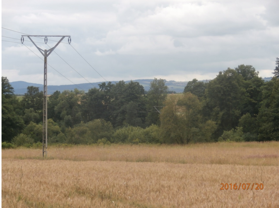
Figure 5 – N-S MV power line in the area of reservoir basin.
