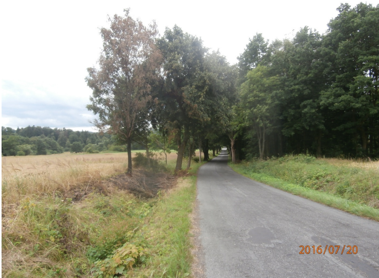
Figure 8 – Section of district road No. 3233D located in the area of the right bank abutment of the dam, western view.
