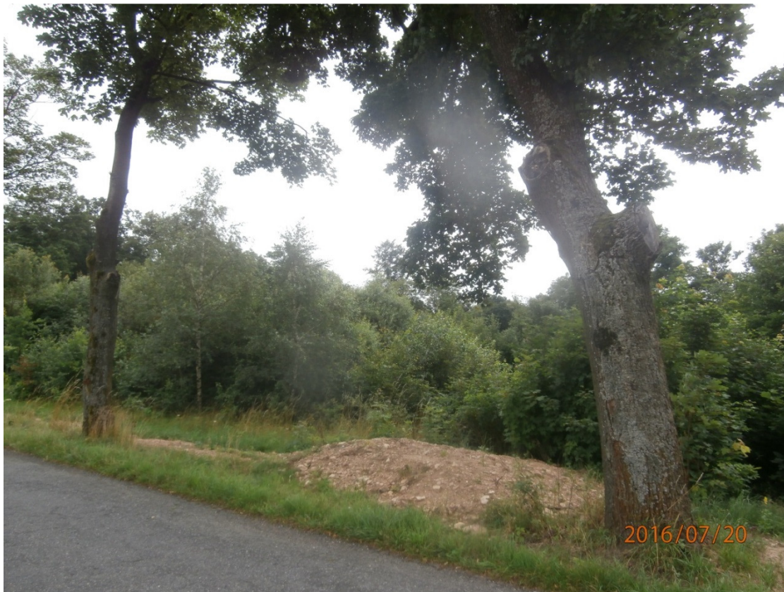
Figure 3 –View from the existing district road No. 3233D on the plot No. 242/5 (indented disassembly of existing foundations).
